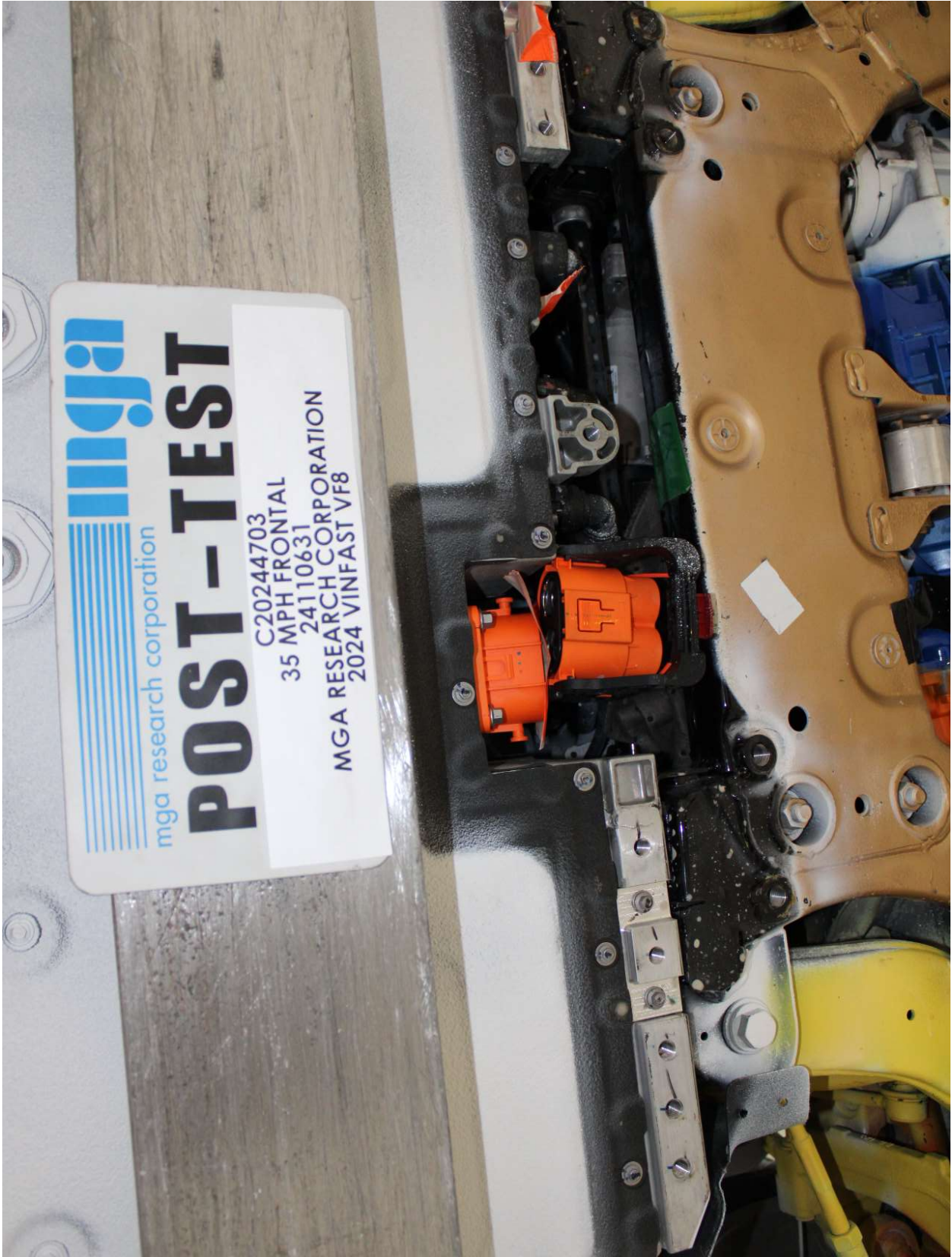
Photo No. 73. Post-Test Voltage Monitoring Leads Attached to Electric Energy Storage System
