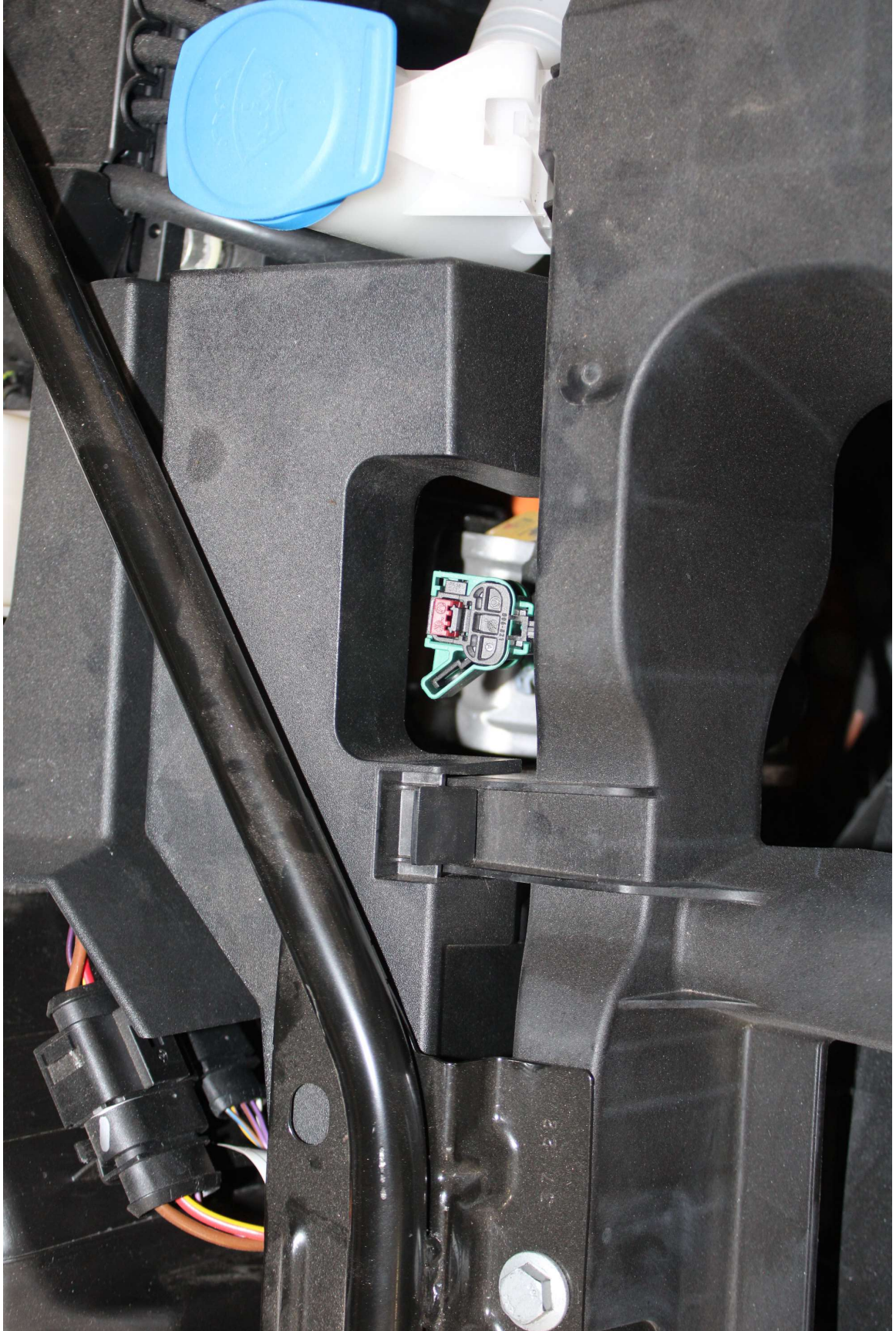
Photo No. 68. Pre-Test Manual Service Disconnect in Place
