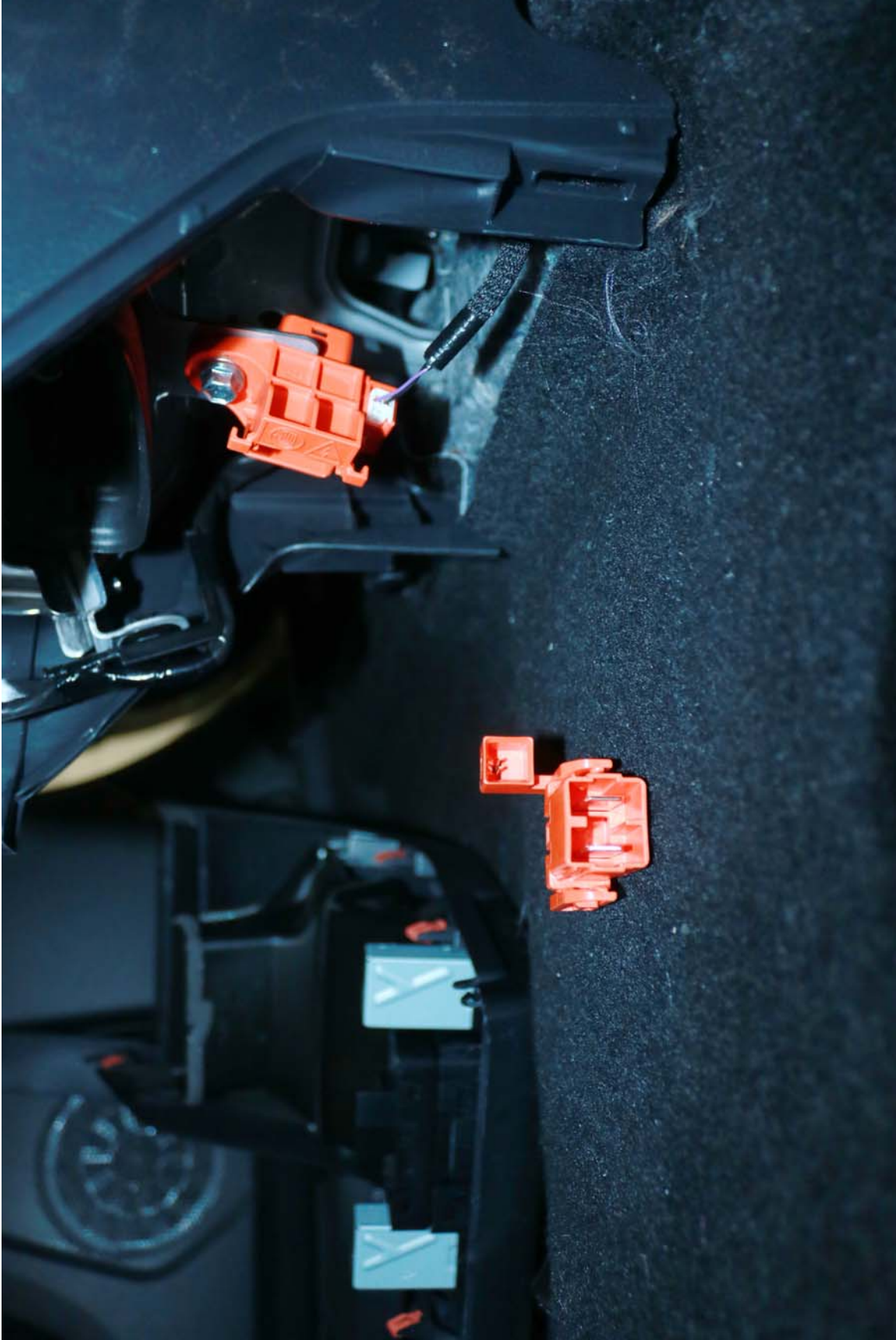
Photo No. 72. Post-Test Manual Service Disconnect Removed
