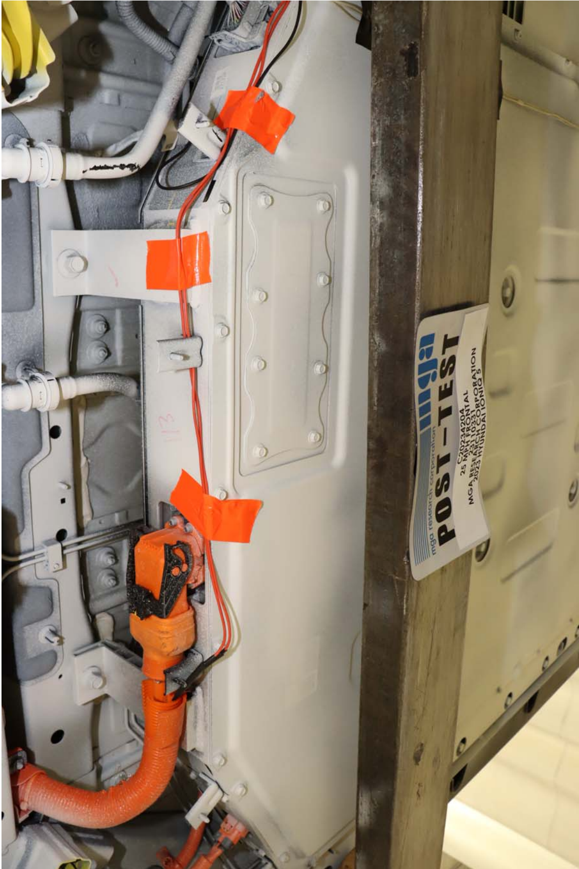
Photo No. 65. Post-Test Voltage Monitoring Leads Attached to Electric Energy Storage System
