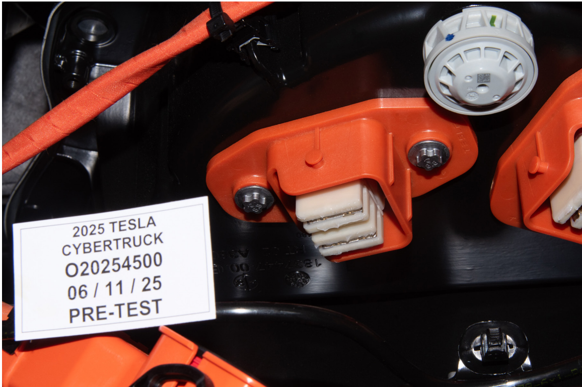
FIGURE 305-08d Manual High Voltage Service Disconnect Removed
