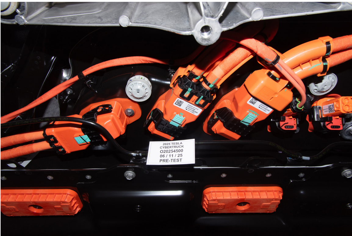
FIGURE 305-06d Manual High Voltage Service Disconnect in Place
