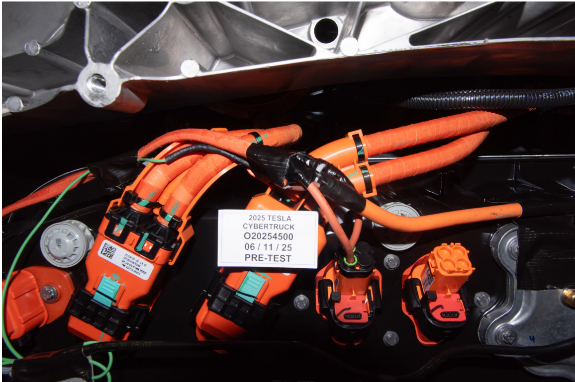
FIGURE 305-022. Pre-Impact View of High Voltage Leads Attached
