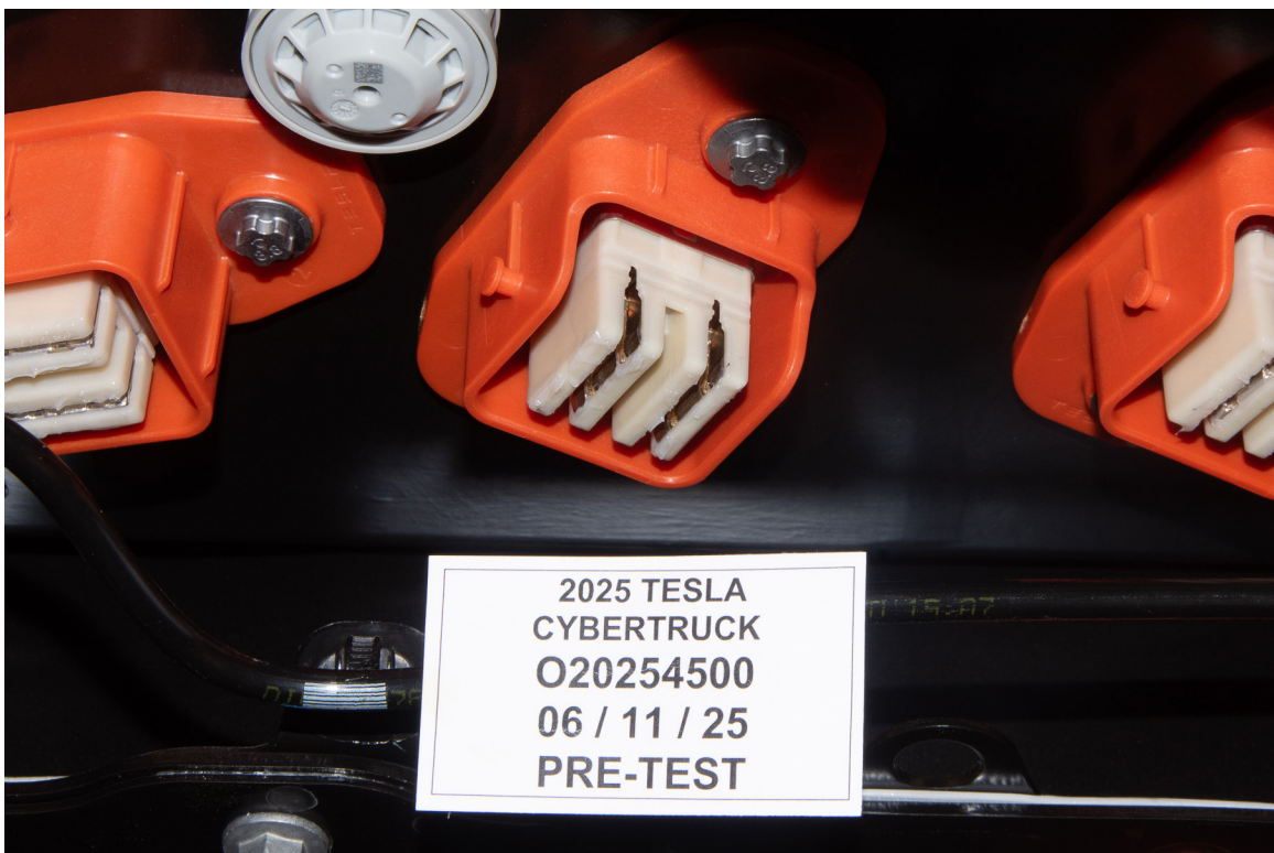
FIGURE 305-08c Manual High Voltage Service Disconnect Removed
