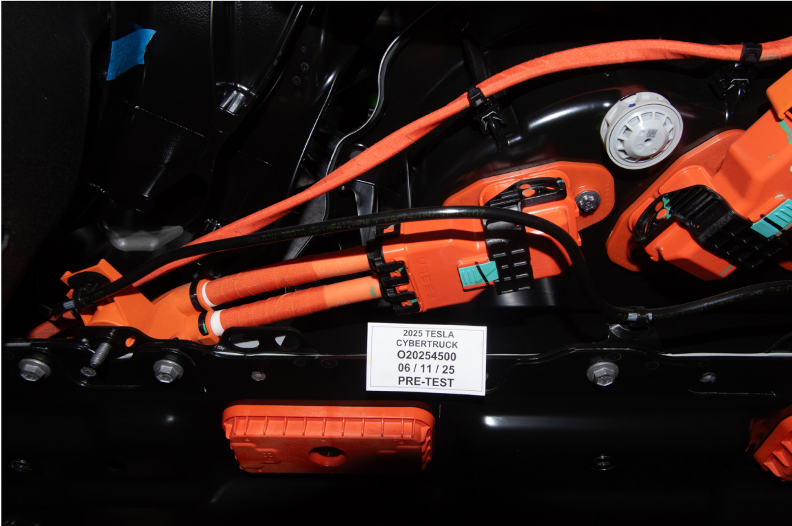
FIGURE 305-06c Manual High Voltage Service Disconnect in Place
