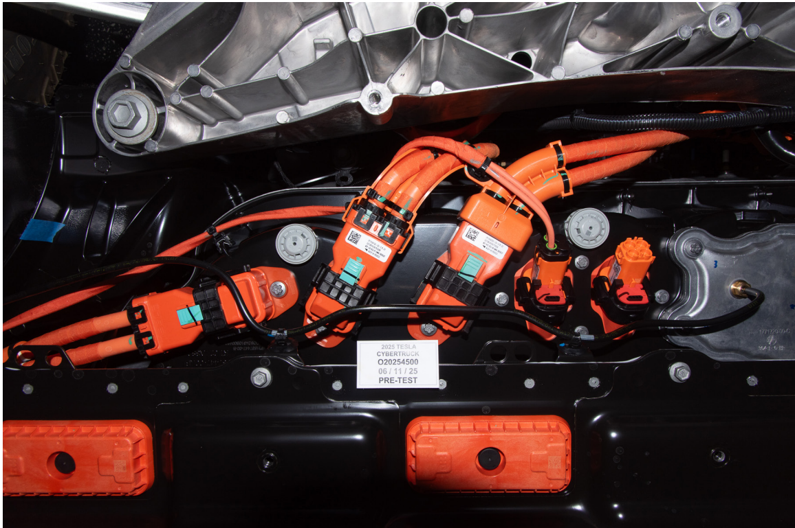
FIGURE 305-06a Manual High Voltage Service Disconnect in Place
