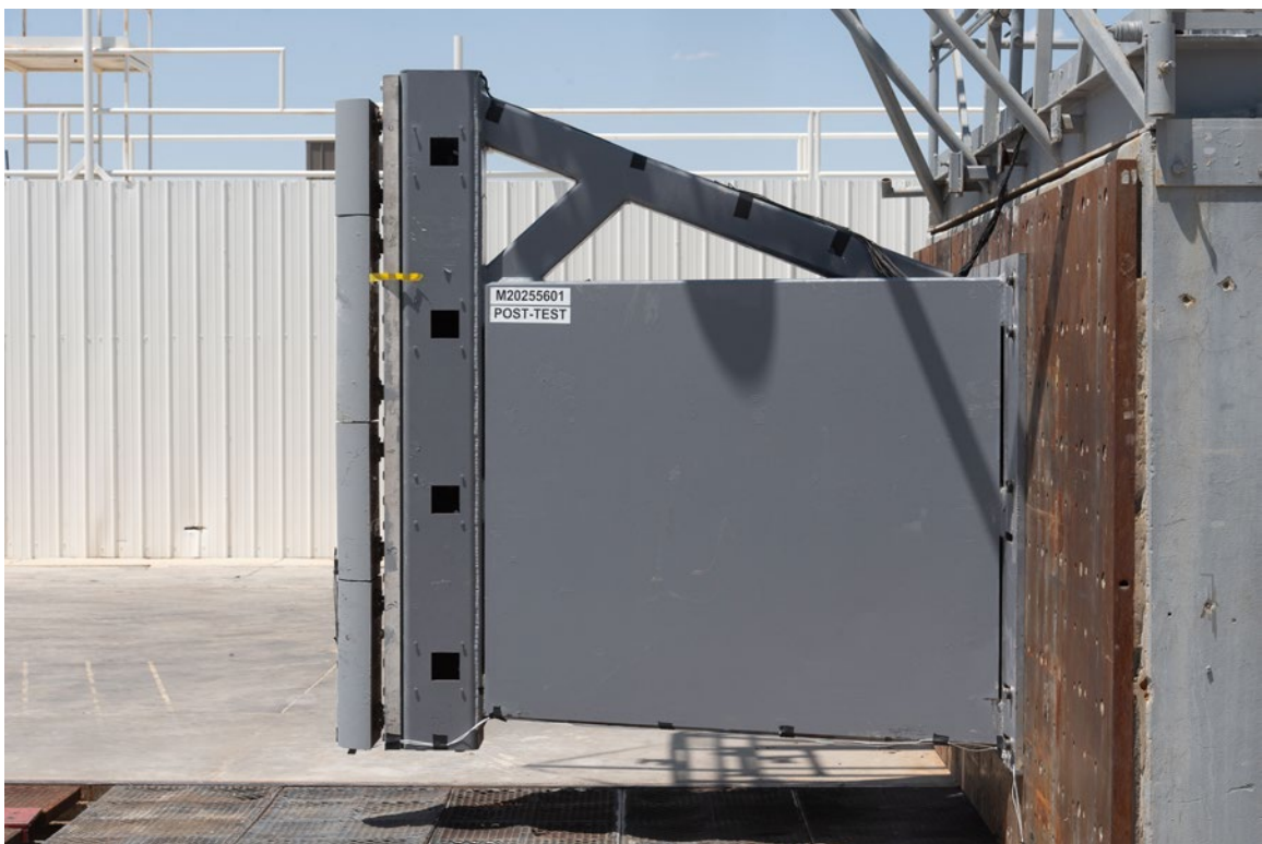
FIGURE 62. Post-Test Pole Barrier Side View
