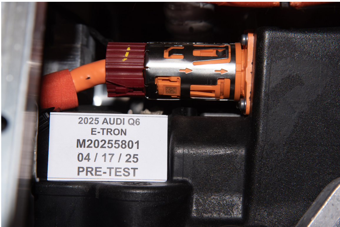
FIGURE 305-018. Pre-Impact View of High Voltage Interconnect(s)
