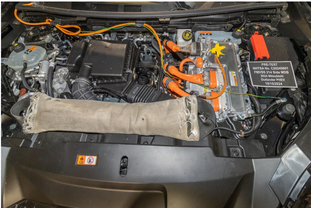
Figure 305-18: Pre-Impact View of High Voltage Interconnects
