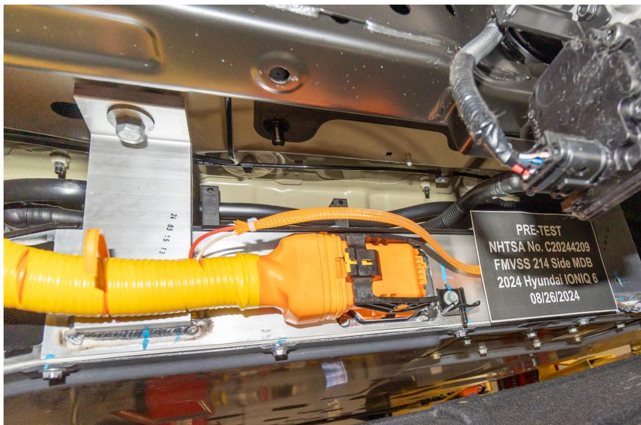
Figure 305-22: Pre-Impact View of High Voltage Leads Attached
