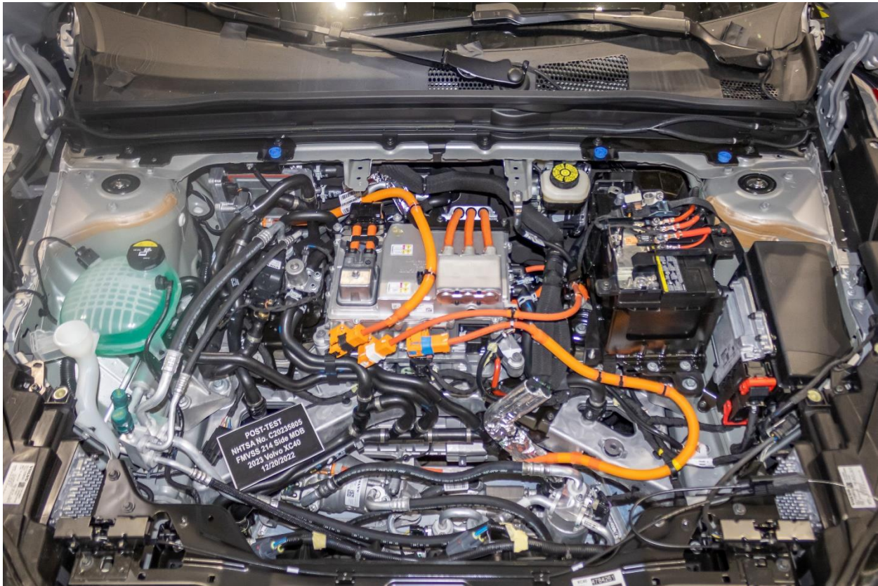
Figure 305-17: Post-Impact View of Electric Propulsion Drive
