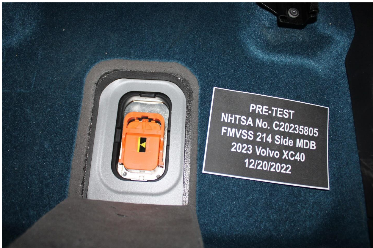
Figure 305-6: Manual High Voltage Service Disconnect in Place
