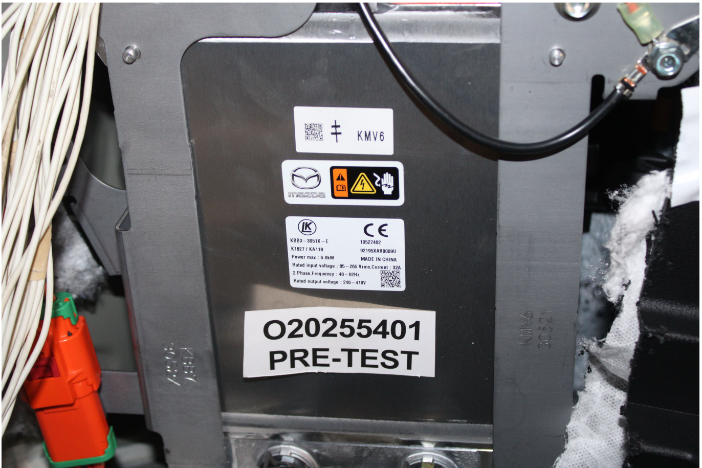
Photo No. 305-05 - Other Vehicle Label(s) Related to Electrical Propulsion System
