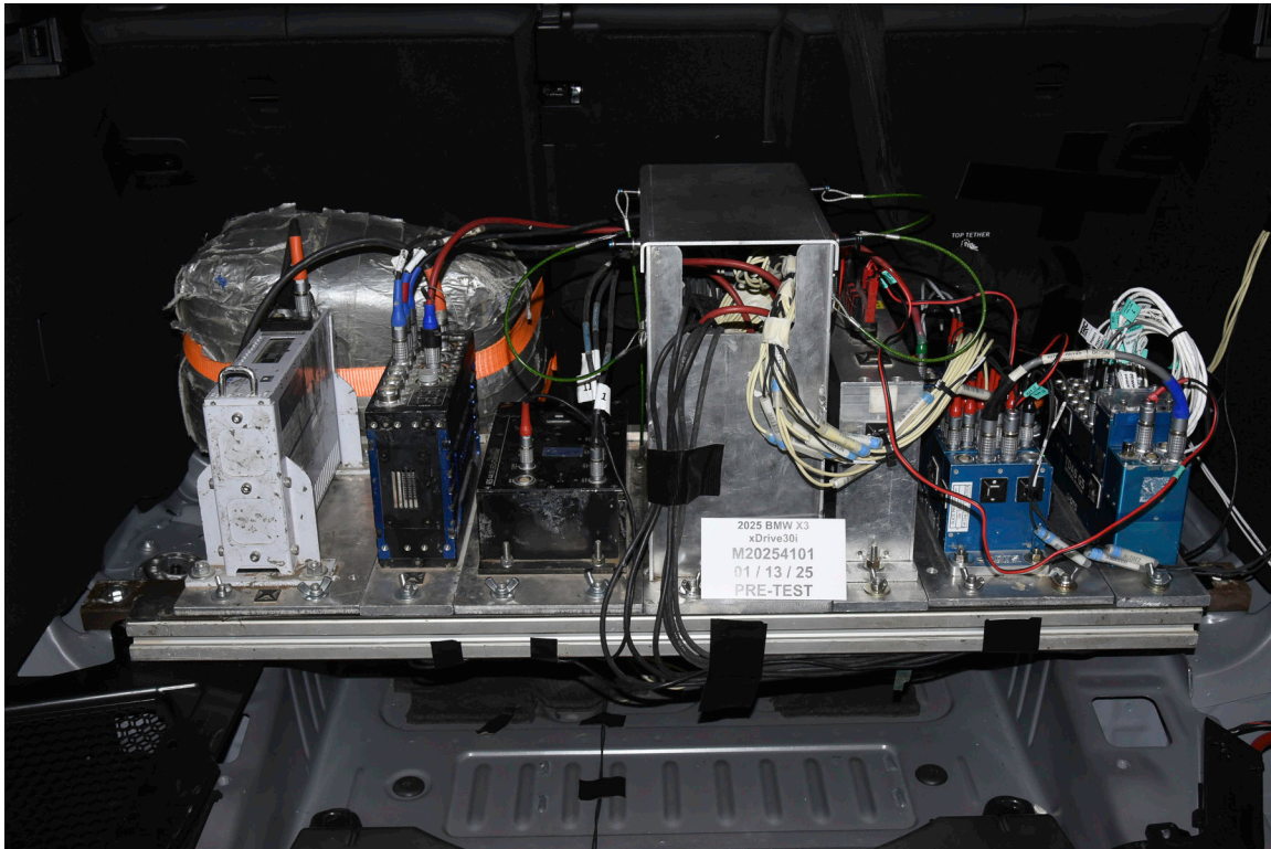
FIGURE 63. Pre-Test Ballast View
