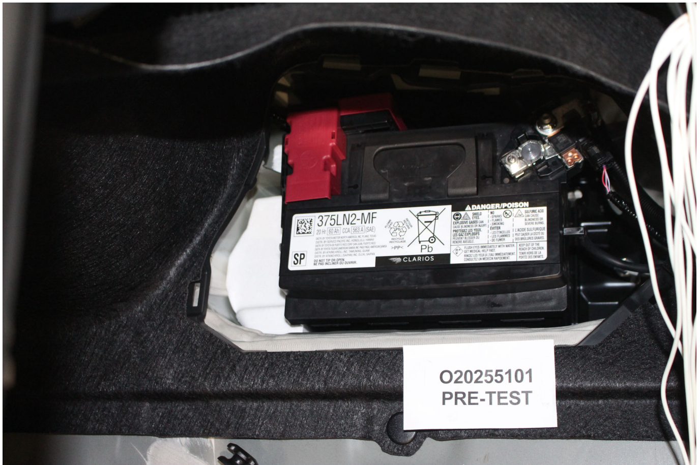
Photo No. 305-01 - Auxiliary Power Module Warning Label
