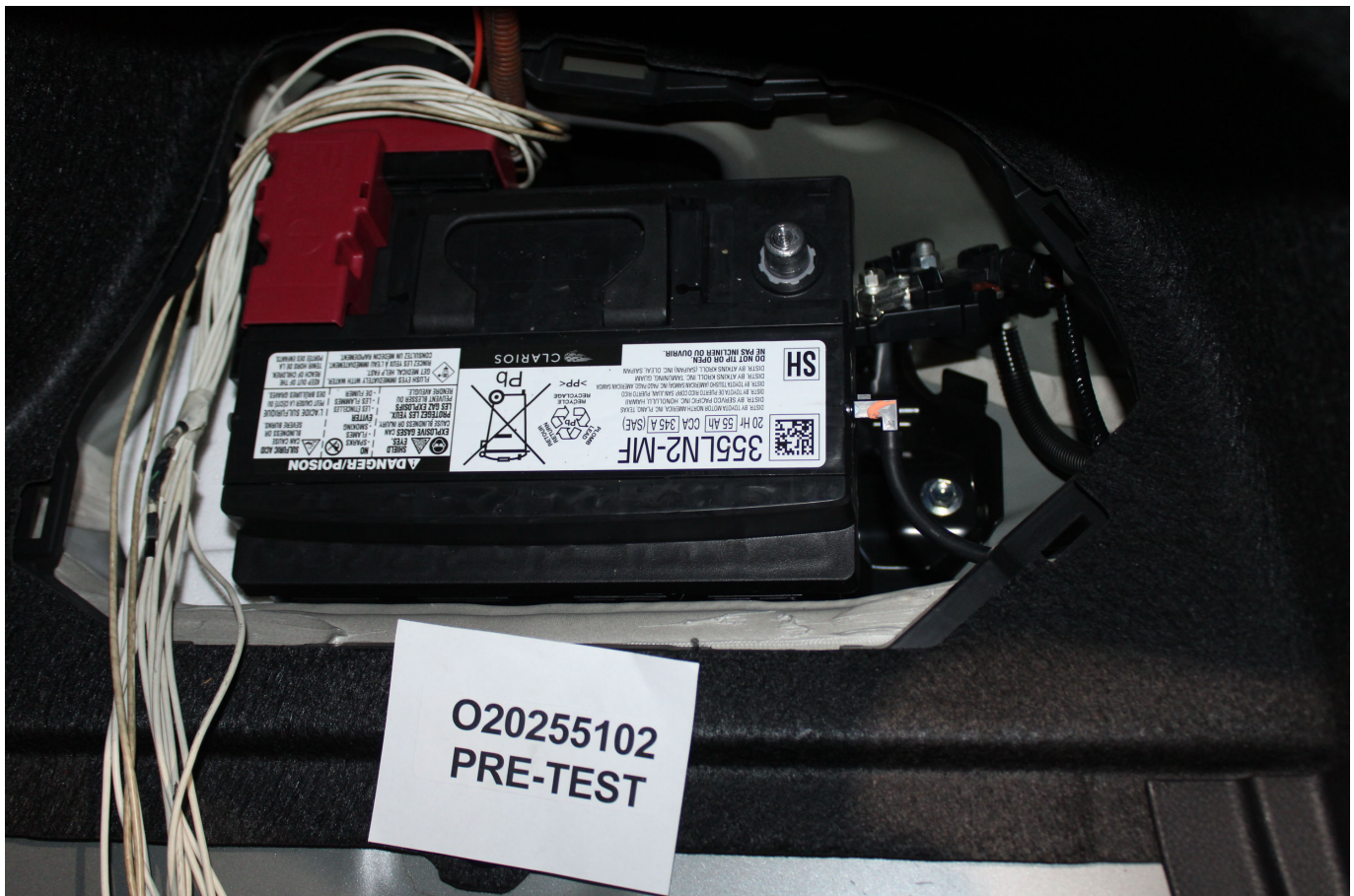
Photo No. 305-01 - Auxiliary Power Module Warning Label
