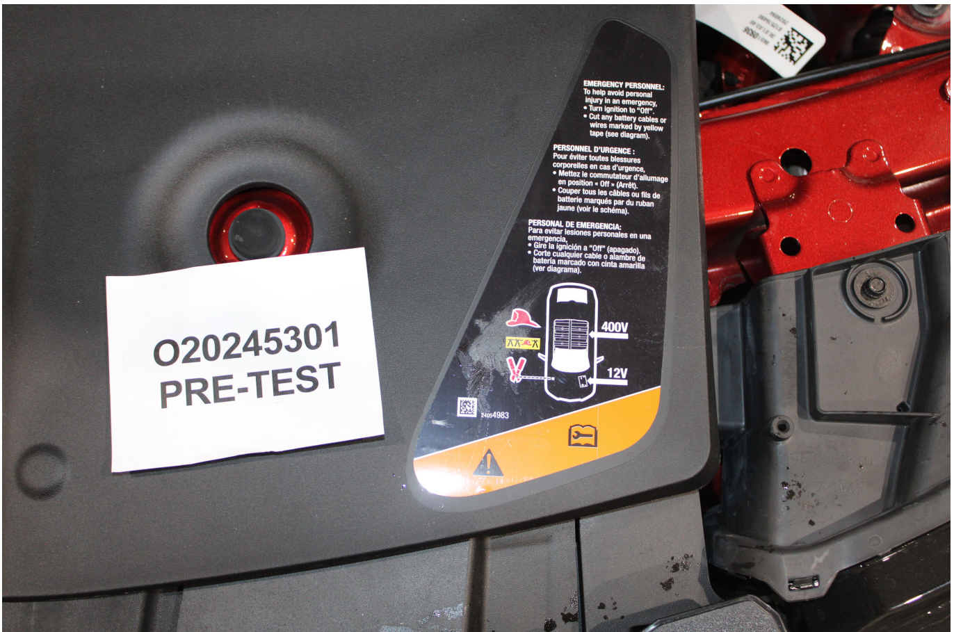
Photo No. 305-03 - First Responder Warning Label
