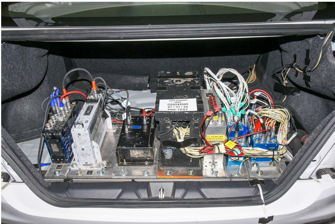
FIGURE 94. Pre-Test Ballast View
