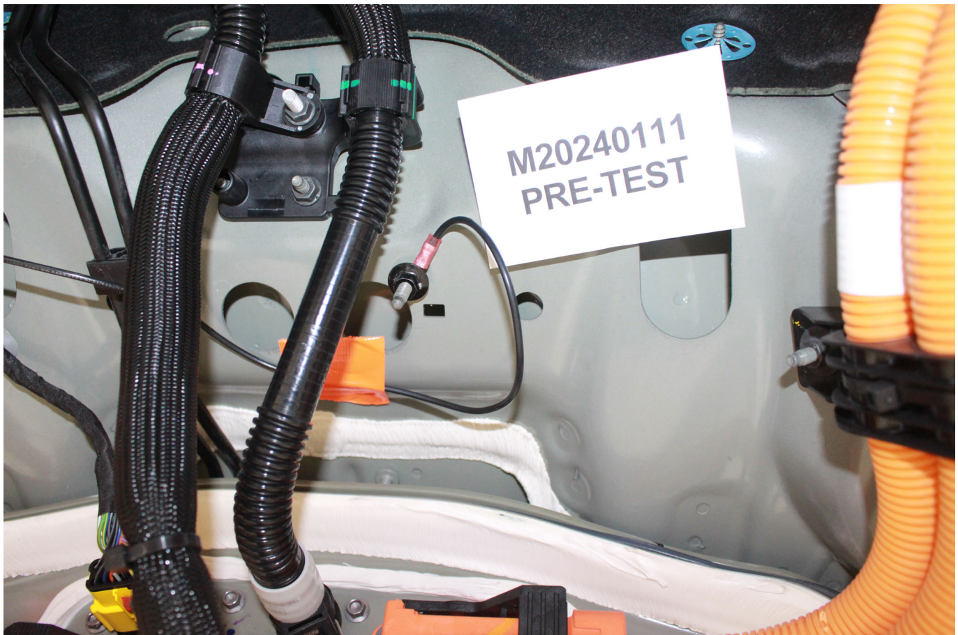
Photo No. 305-21 - Pre-Impact View of Ground Lead Attached
