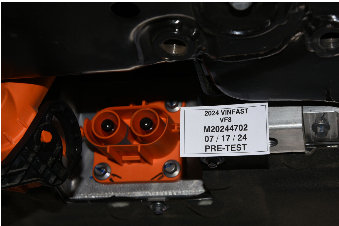
FIGURE 305-08 Manual High Voltage Service Disconnect Removed
