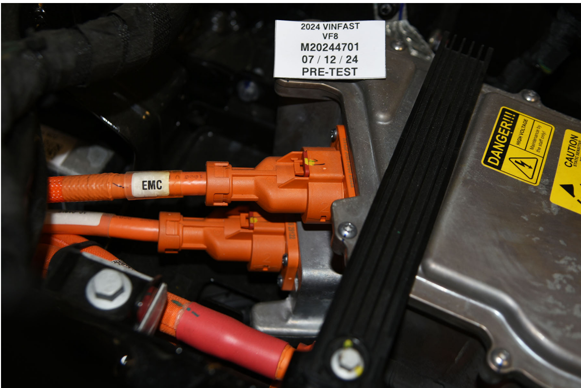
FIGURE 305-019 Pre-Impact View Propulsion Battery Venting System(s)
