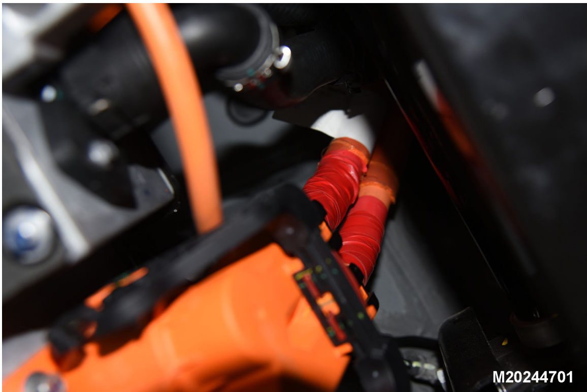
FIGURE 305-023 Pre-Impact Close-Up View of High Voltage Leads Attached
