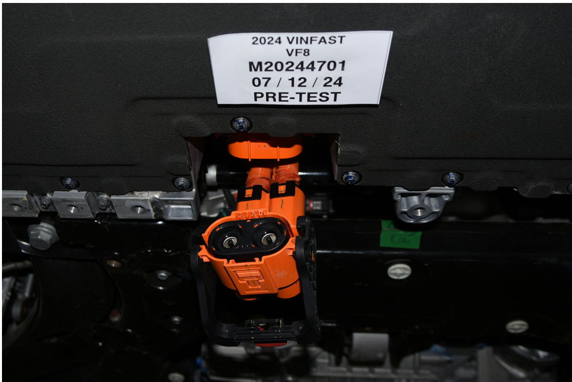
FIGURE 305-07 Manual High Voltage Service Disconnect Removed
