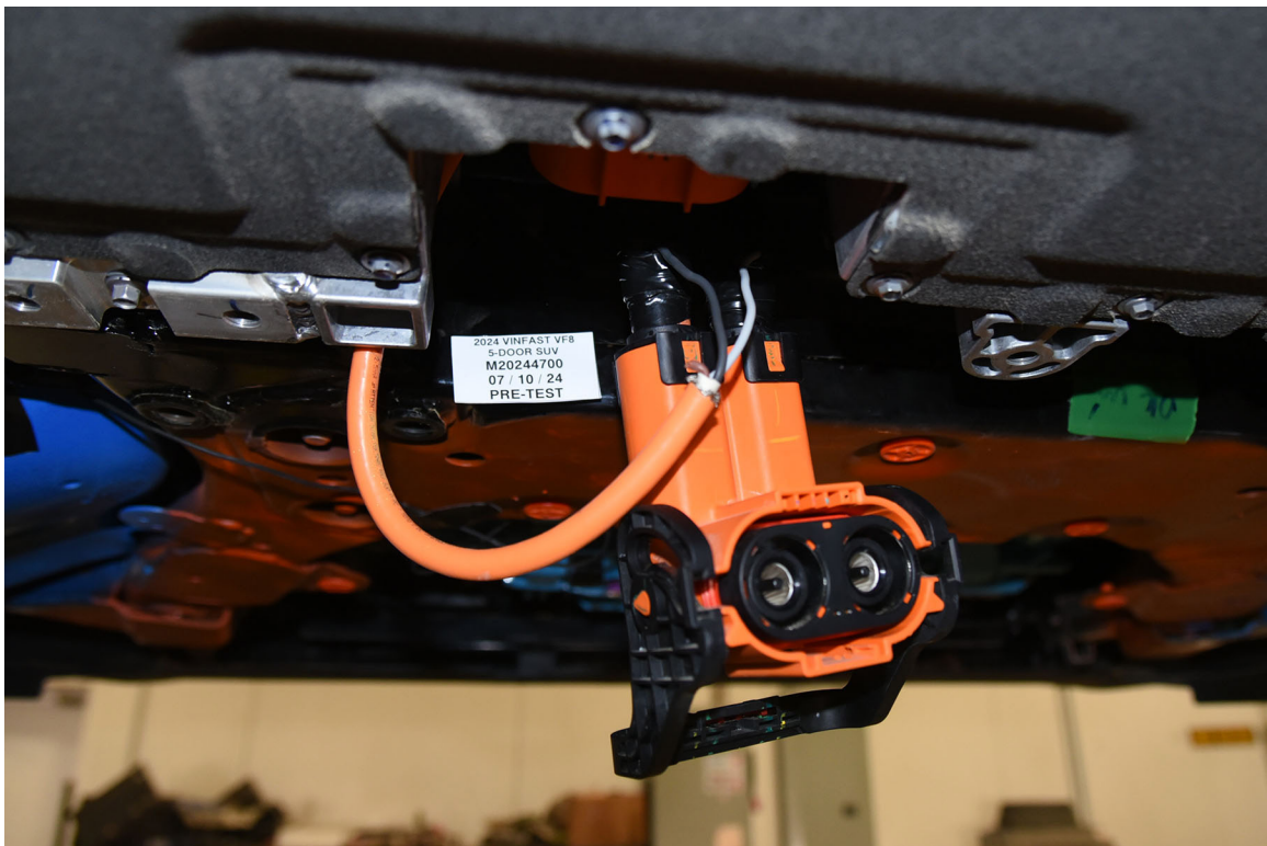
FIGURE 305-07 Manual High Voltage Service Disconnect Removed
