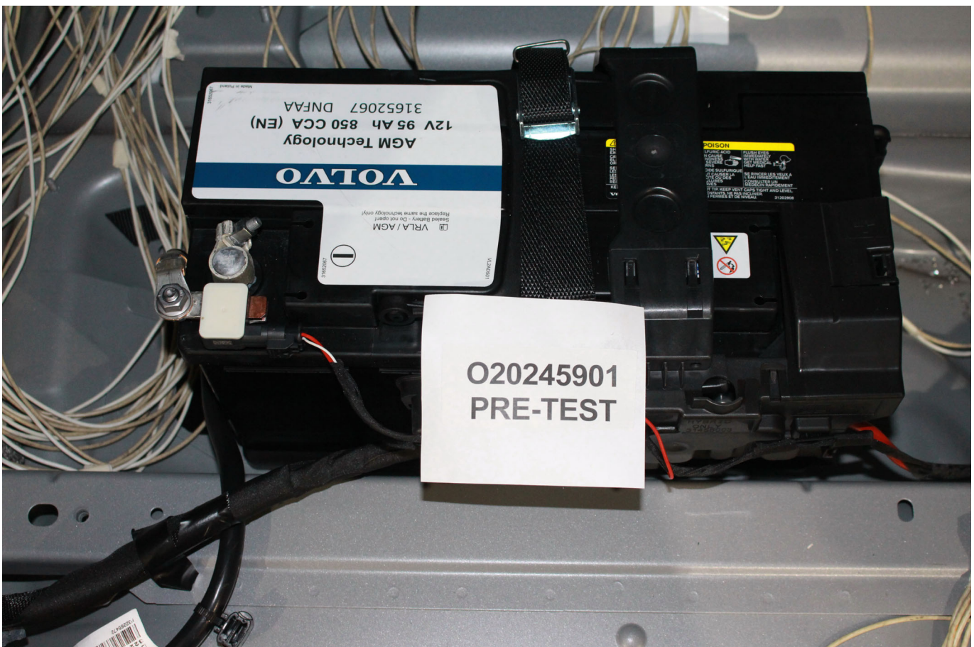
Photo No. 305-01 - Auxiliary Power Module Warning Label
