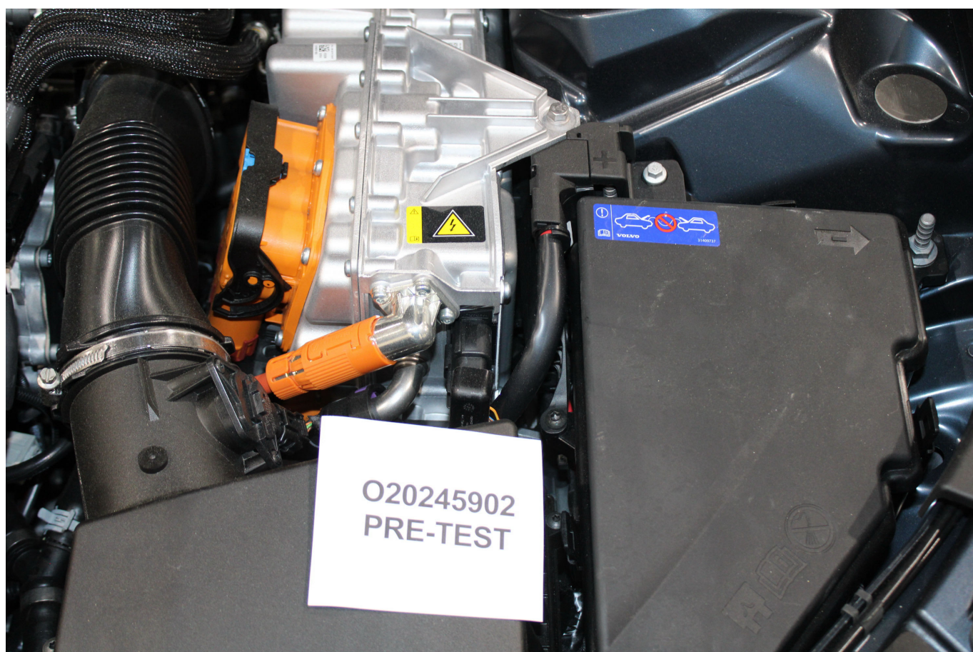
Photo No. 305-02 - Power Inverter Warning Label
