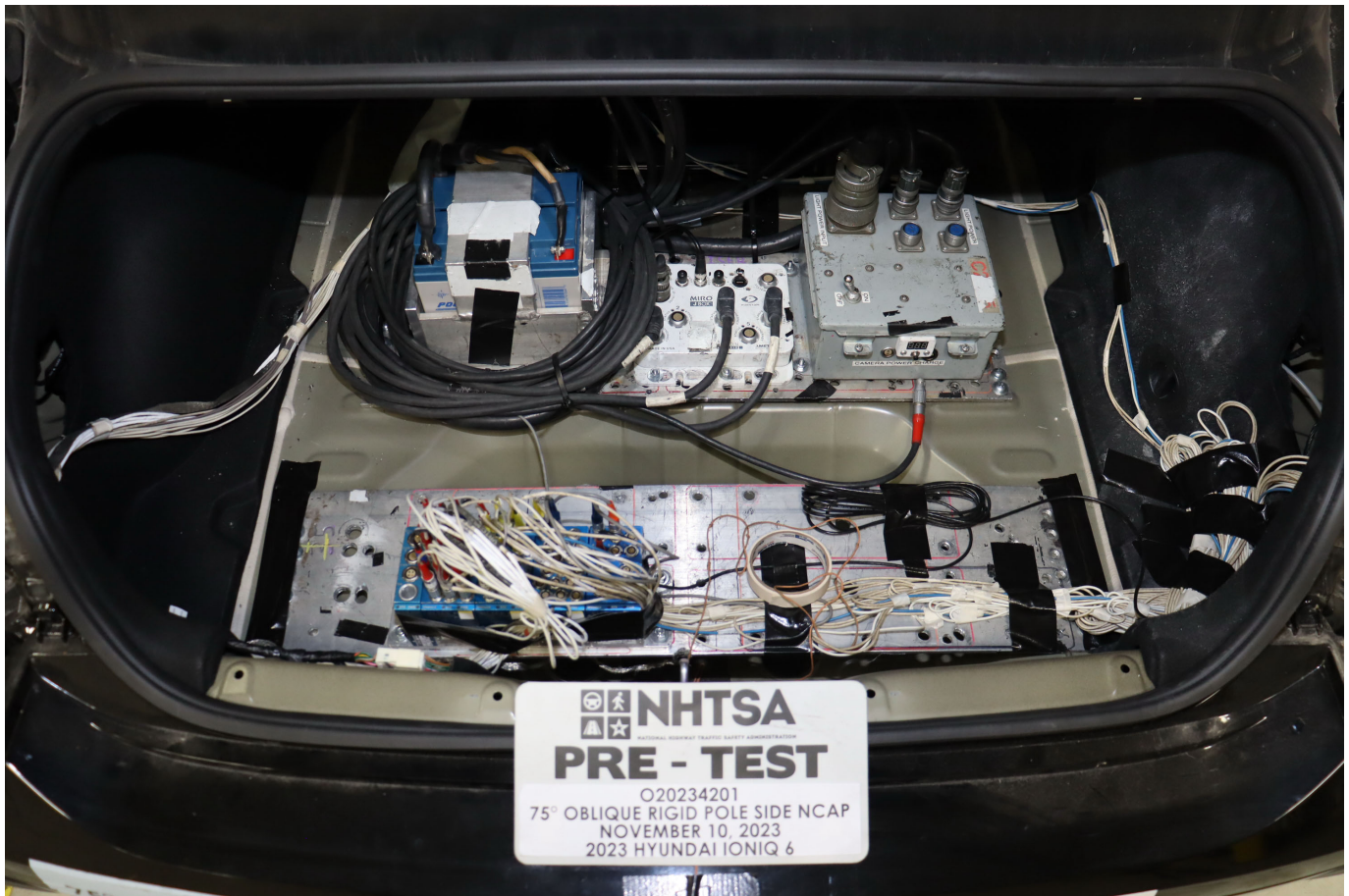
Photo No. 063 - Pre-Test Ballast View
