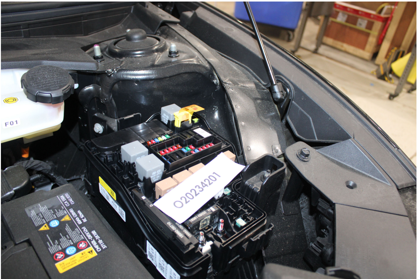
Photo No. 305-04 - First Responder Warning Location
