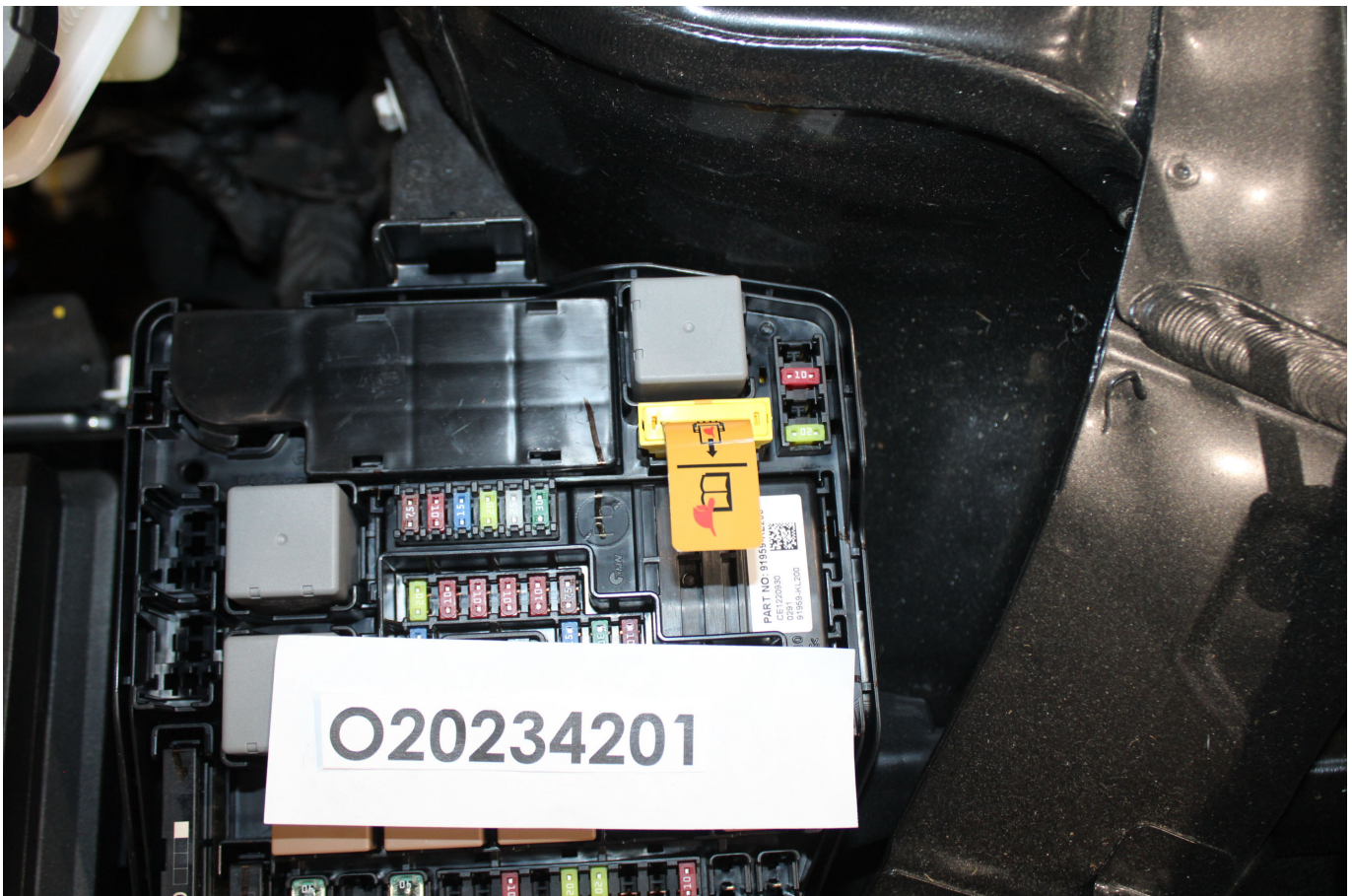
Photo No. 305-03 - First Responder Warning Label
