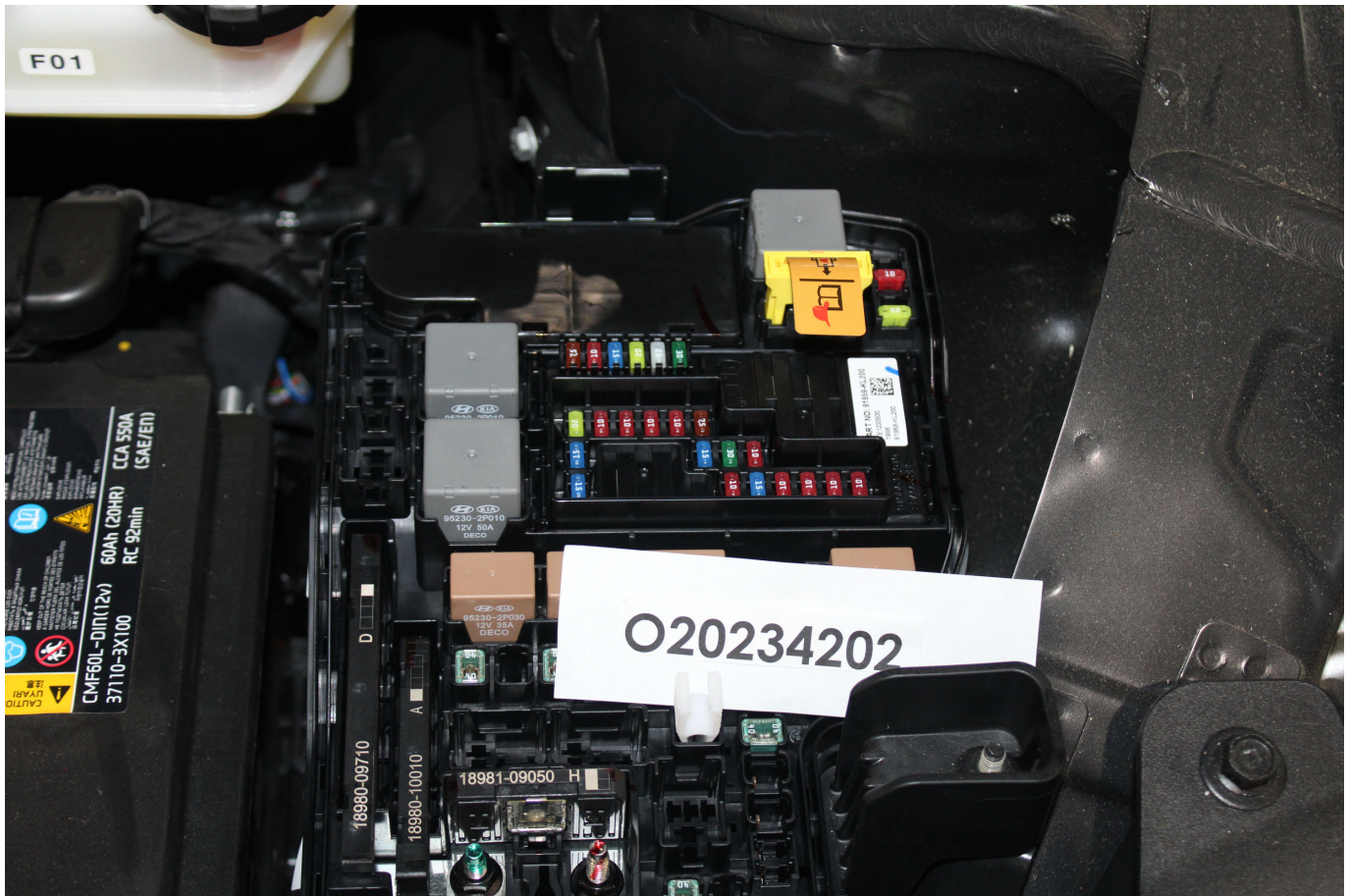
Photo No. 305-03 - First Responder Warning Label
