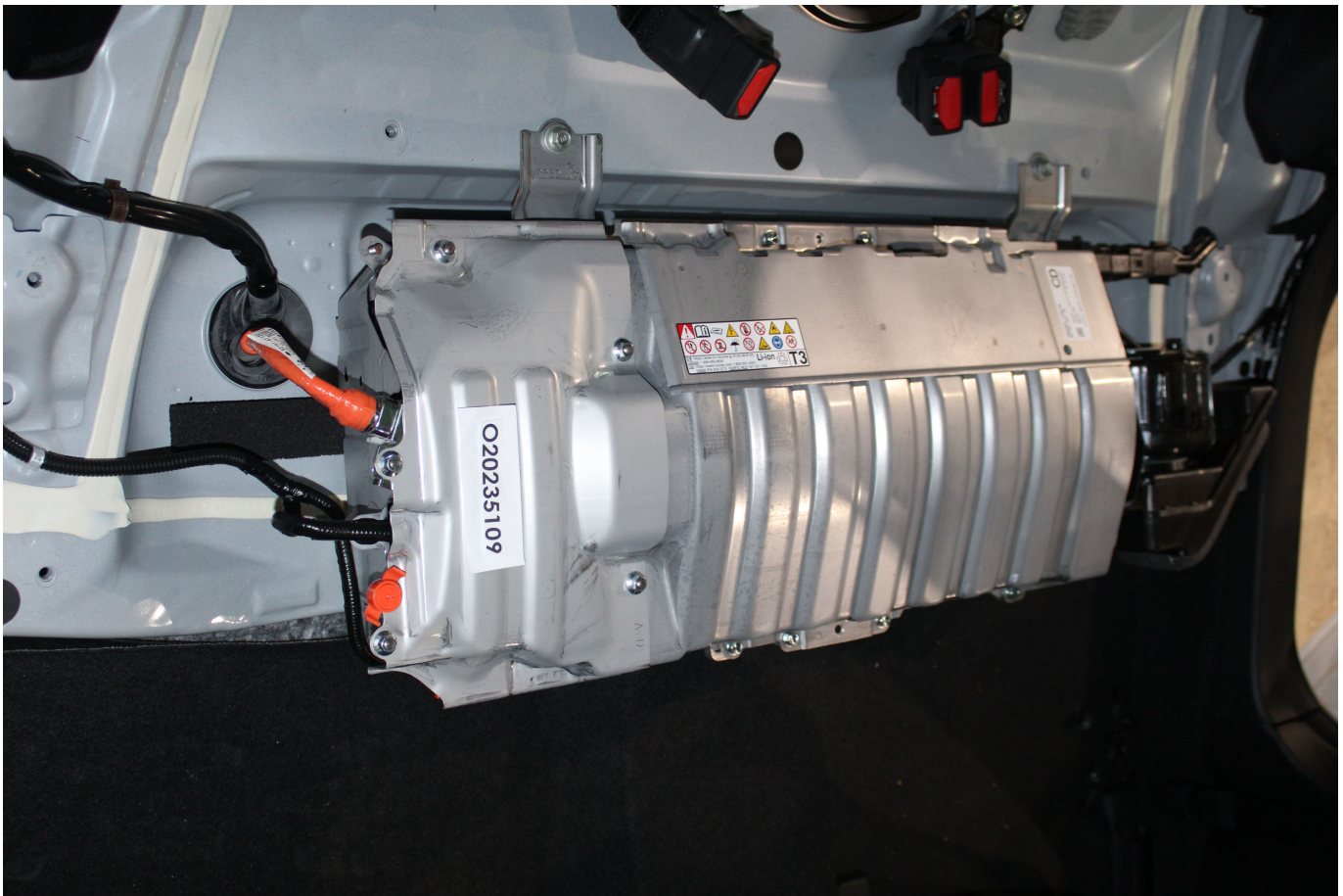
Photo No. 305-09 - Pre-Impact View of Propulsion Battery
