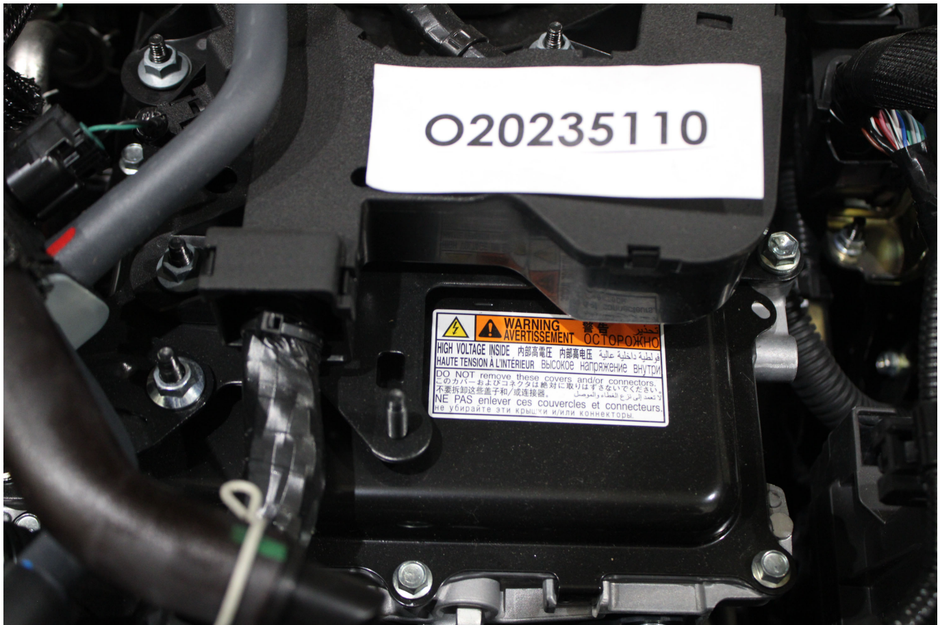
Photo No. 305-02 - Power Inverter Warning Label
