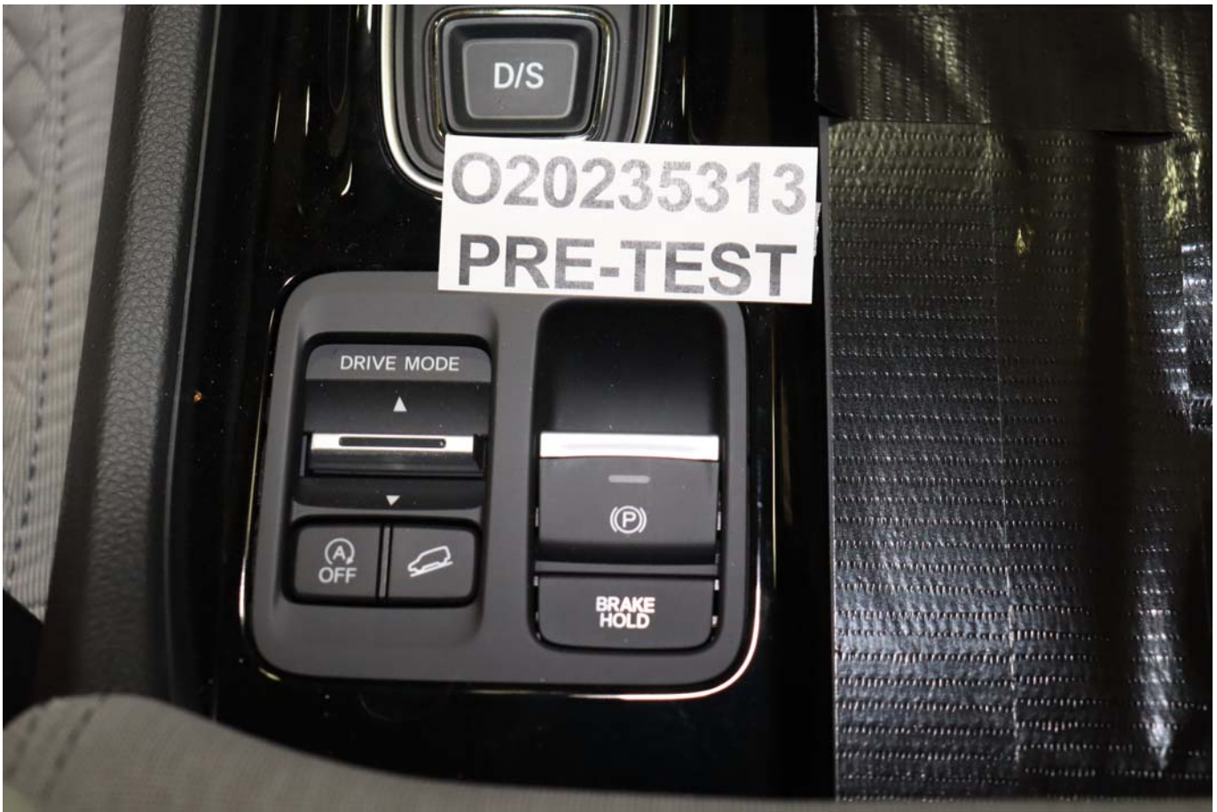
Photo No. 035 - Pre-Test View of Disengaged Parking Brake
