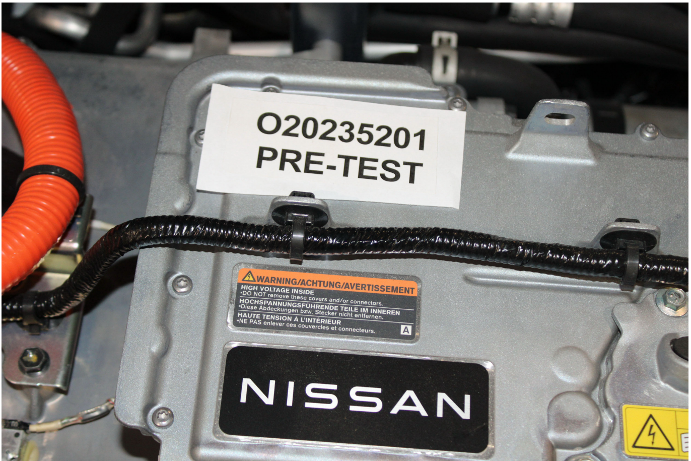
Photo No. 305-02 - Power Inverter Warning Label
