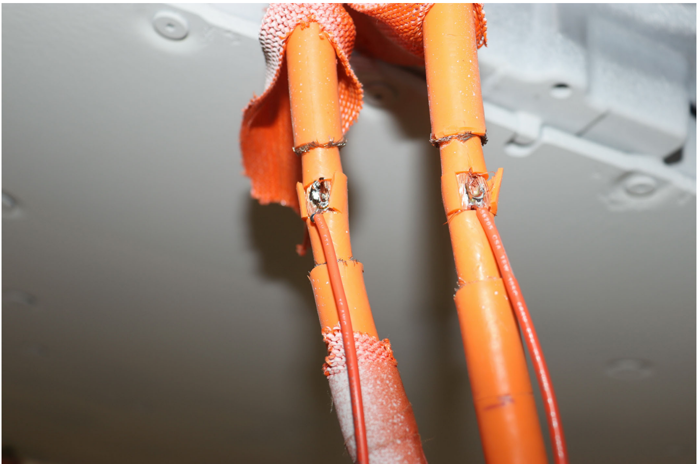
Photo No. 305-23 - Pre-Impact Close-Up View of High Voltage Leads Attached
