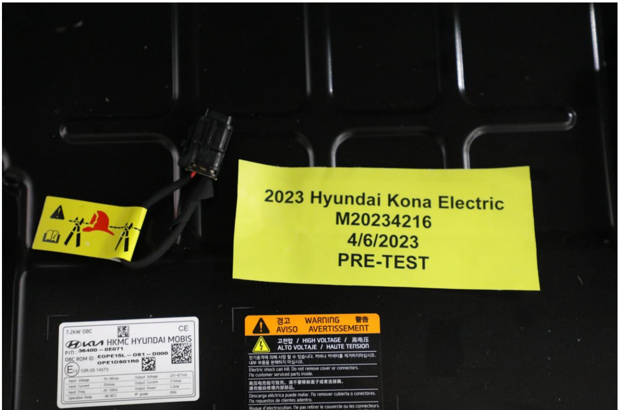
305-07 Manual High Voltage Service Disconnect Removed
