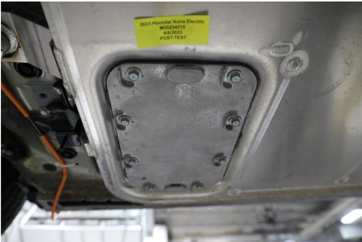
305-13 Post-Impact View of Battery Box(s) or Container(s) Which Holds Individual Battery Modules
