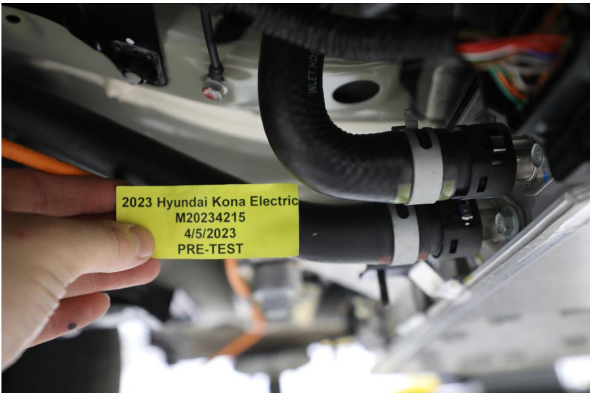
305-19 Pre-Impact View Propulsion Battery Venting System(s)
