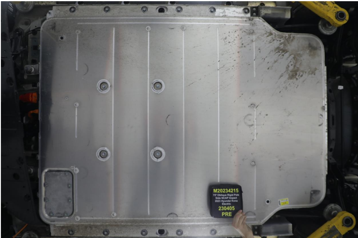
305-09 Pre-Impact View of Propulsion Battery
