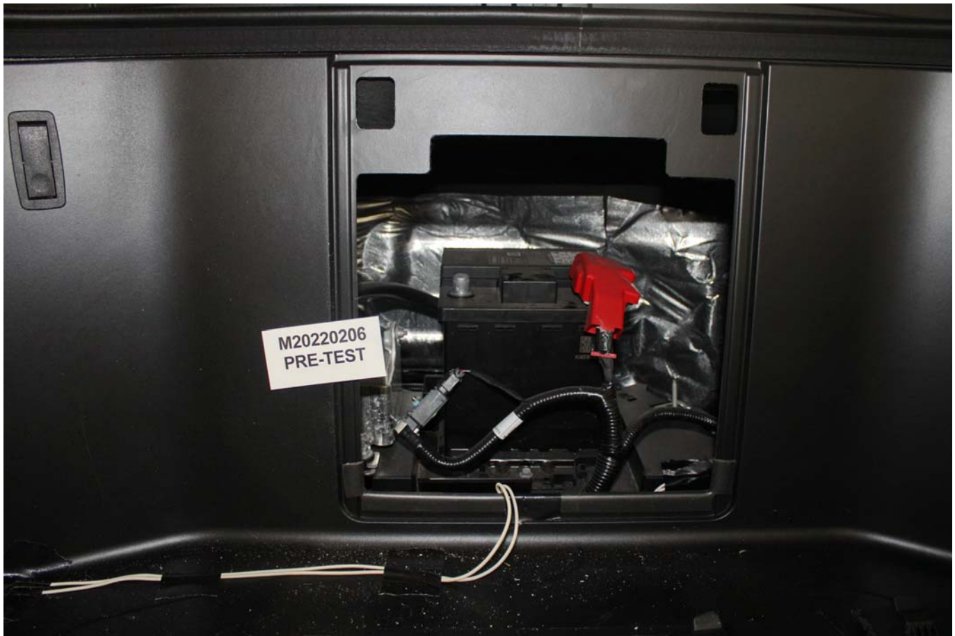
Photo No. 305-01 - Auxiliary Power Module Warning Label
