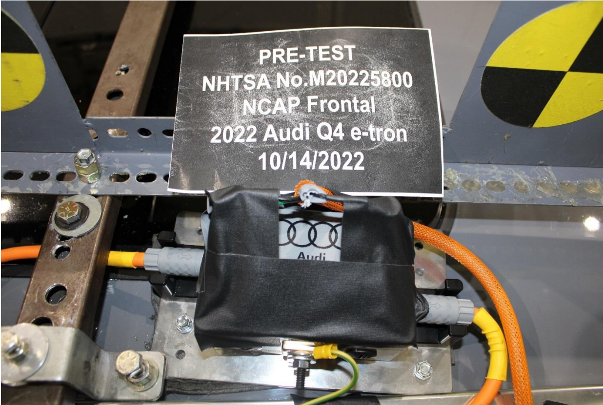
Figure 305-18: Pre-Impact View of High Voltage Interconnects
