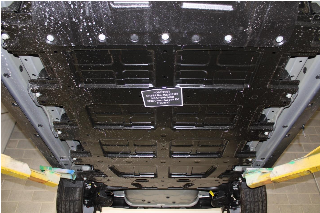
Figure 305-13: Post-Impact View of Battery Box(s) or Container(s) Which Holds Individual Battery Modules
