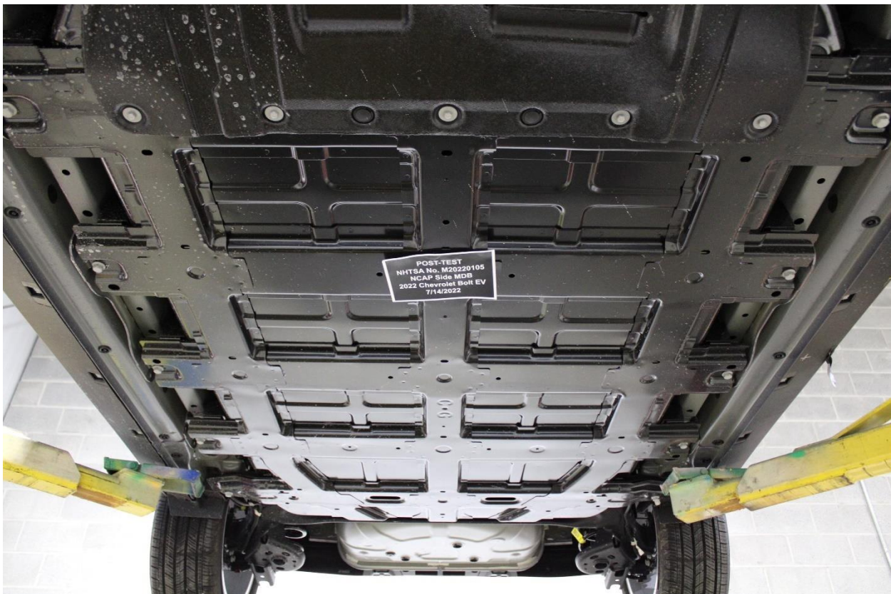
Figure 305-10: Post-Impact Front View of Propulsion Battery
