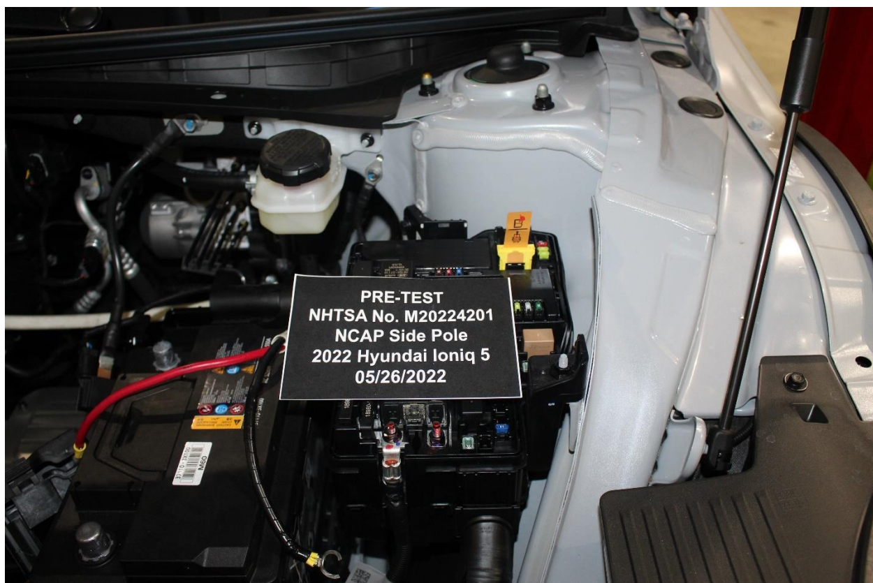
Figure 305-8: Manual High Voltage Service Disconnect Removed Location
