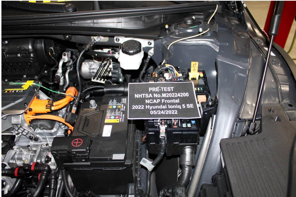
Figure 305-8: Manual High Voltage Service Disconnect Removed Location
