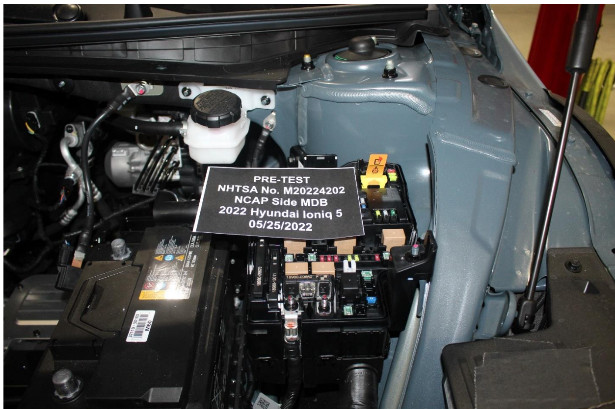
Figure 305-8: Manual High Voltage Service Disconnect Removed Location
