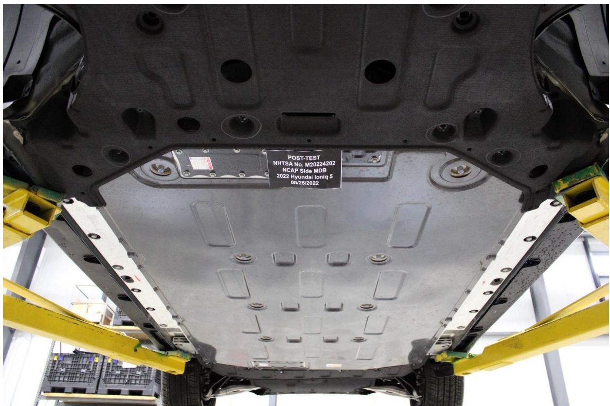
Figure 305-10: Post-Impact Front View of Propulsion Battery
