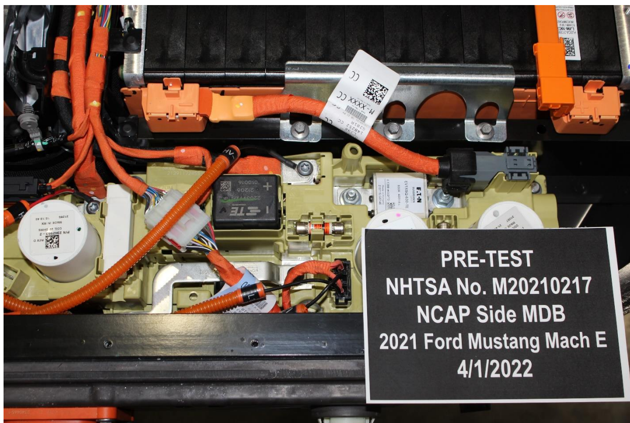
Figure 305-18: Pre-Impact View of High Voltage Interconnects
