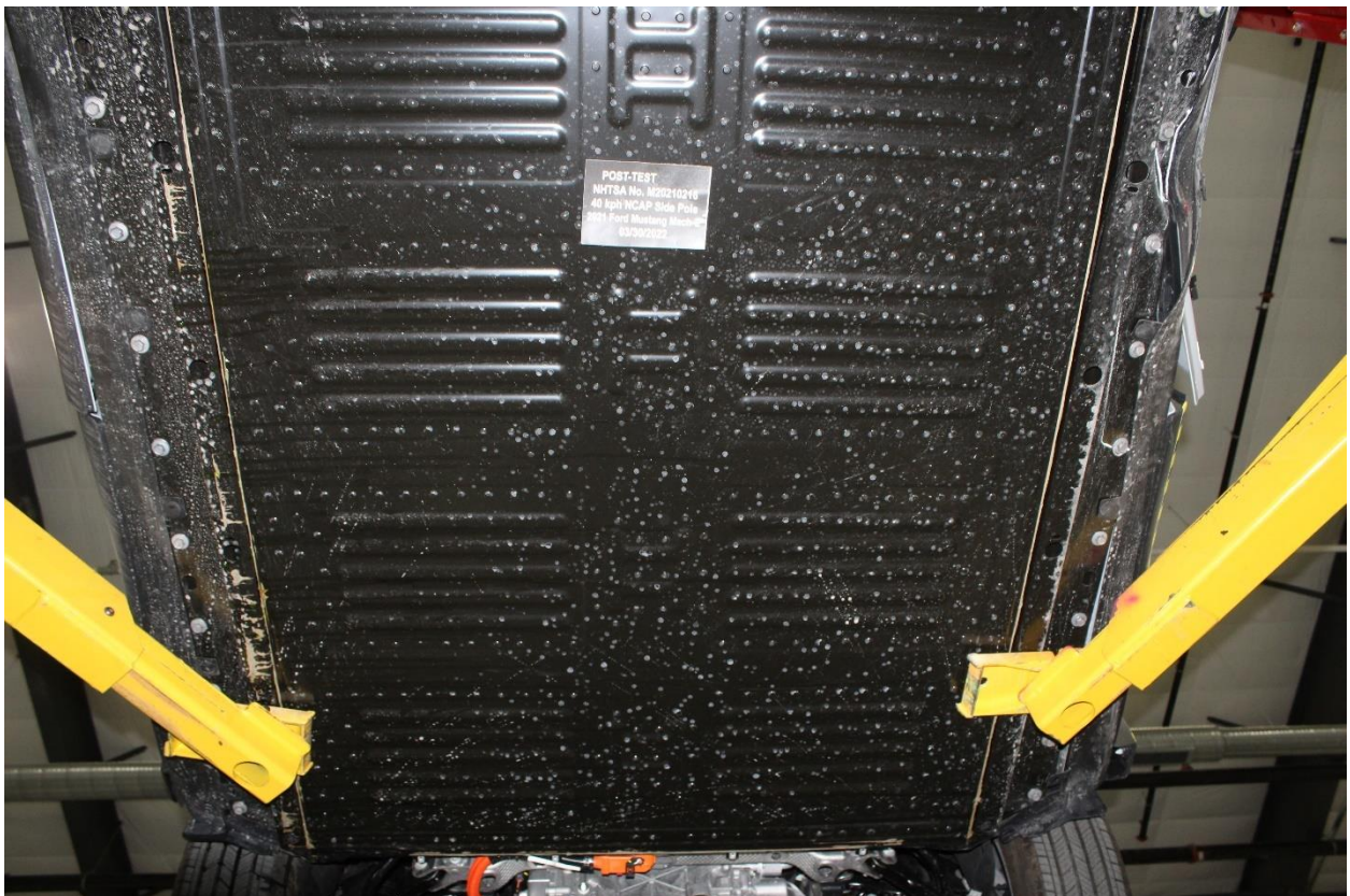
Figure 305-10: Post-Impact Front View of Propulsion Battery
