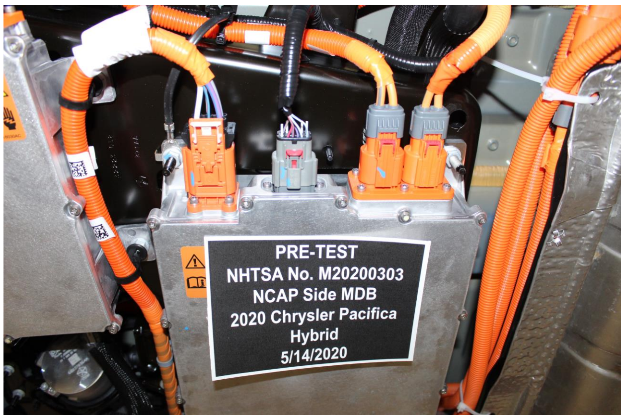
Figure 305-18: Pre-Impact View of High Voltage Interconnects
