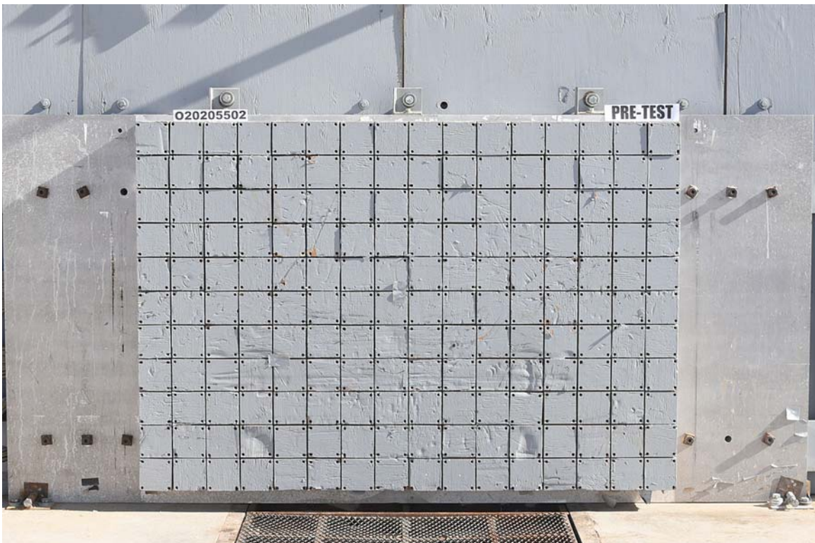
FIGURE 2. Pre-Test Load Cell Wall
