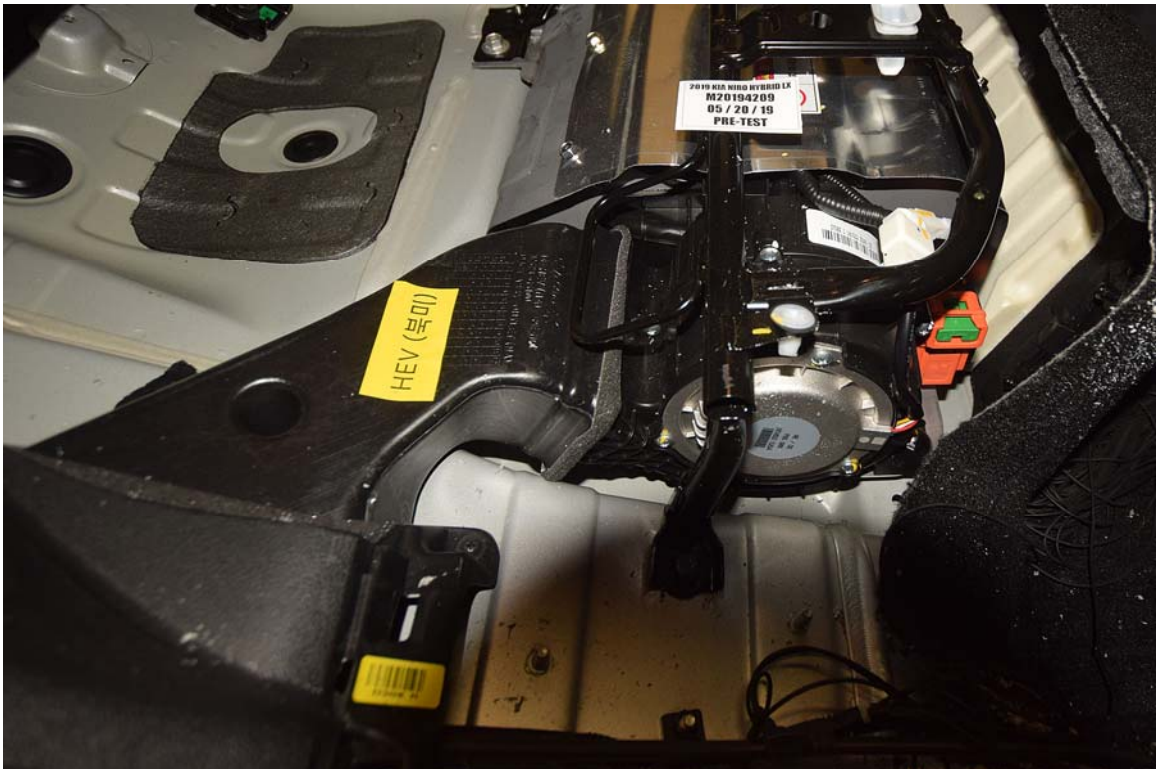
FIGURE 19. Pre-Impact View Propulsion Battery Venting System(s)
