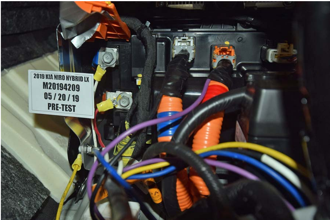
FIGURE 23. Pre-Impact Close-Up View of High Voltage Leads Attached
