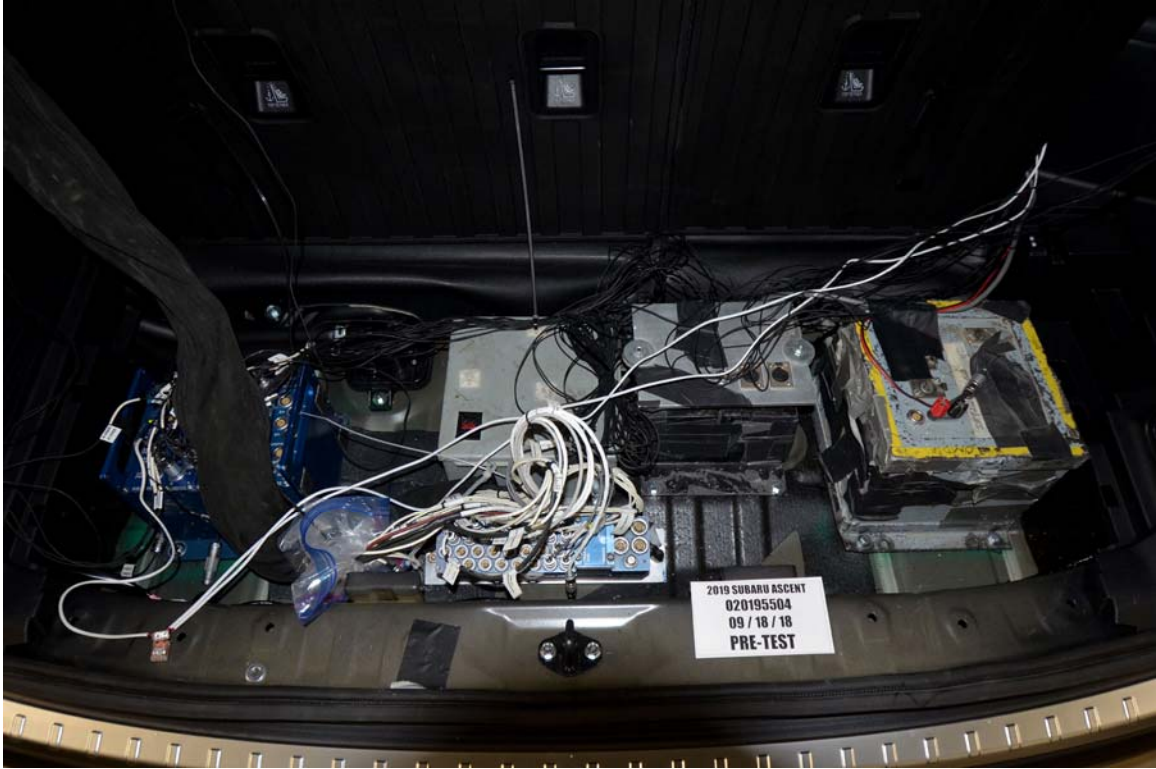
FIGURE 61. Pre-Test Ballast View
