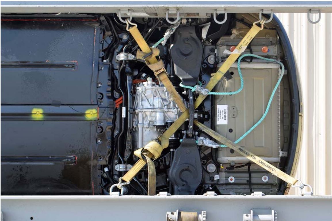
FIGURE 12. Post-Impact Rear View of Propulsion Battery
