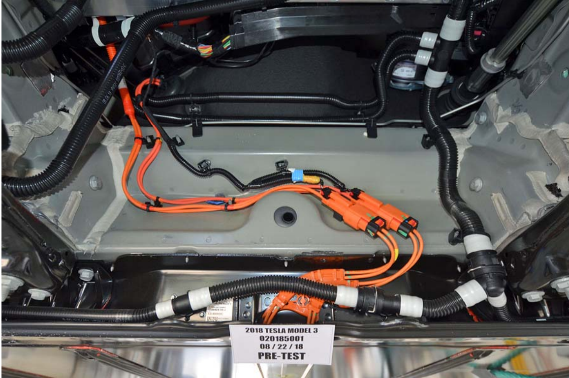
FIGURE 19. Pre-Impact View of High Voltage Interconnect(s)
