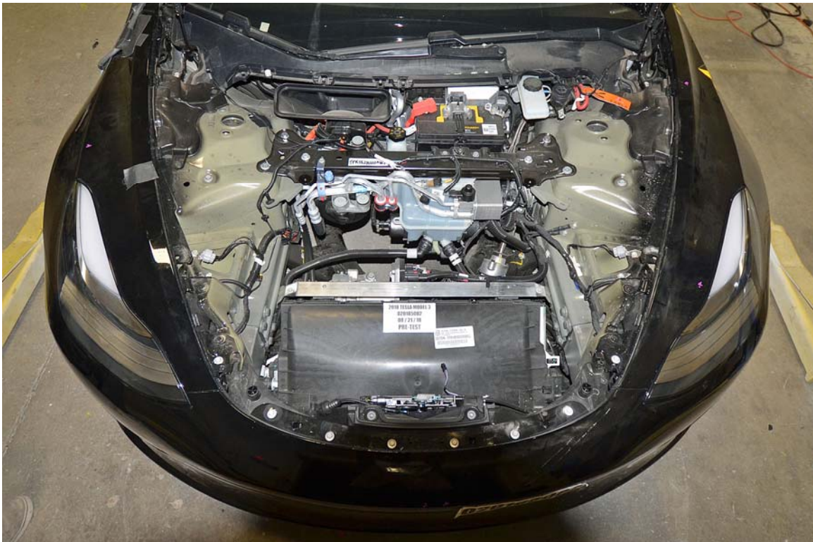
FIGURE 20. Pre-Impact View of Propulsion Battery Venting System(s)
