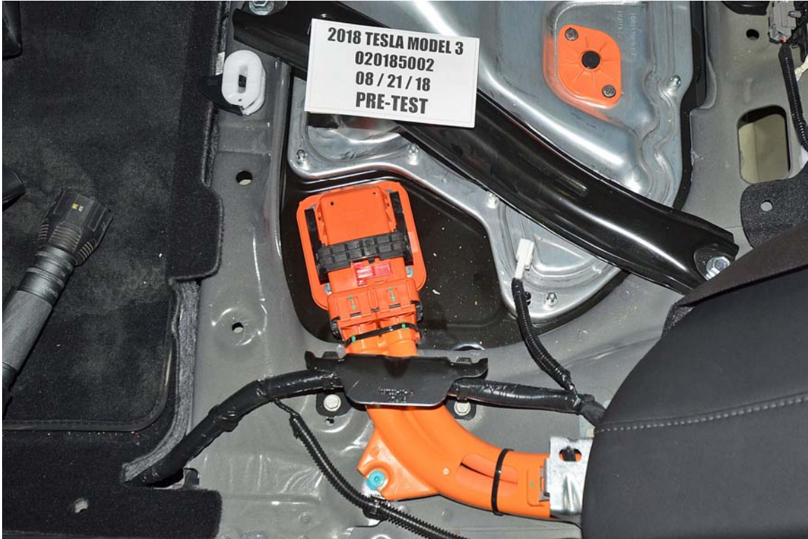
FIGURE 19. Pre-Impact View of High Voltage Interconnect(s)
