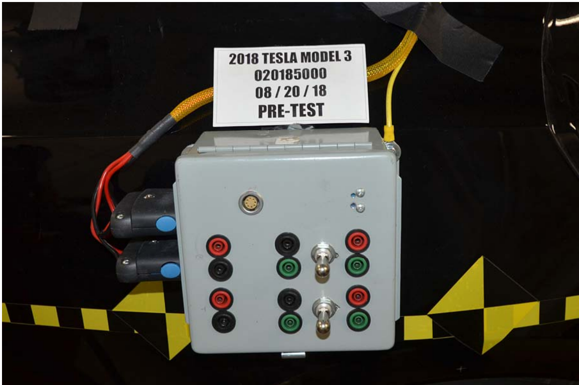
FIGURE 25. Pre-Impact View of Installed Test Interface Port
