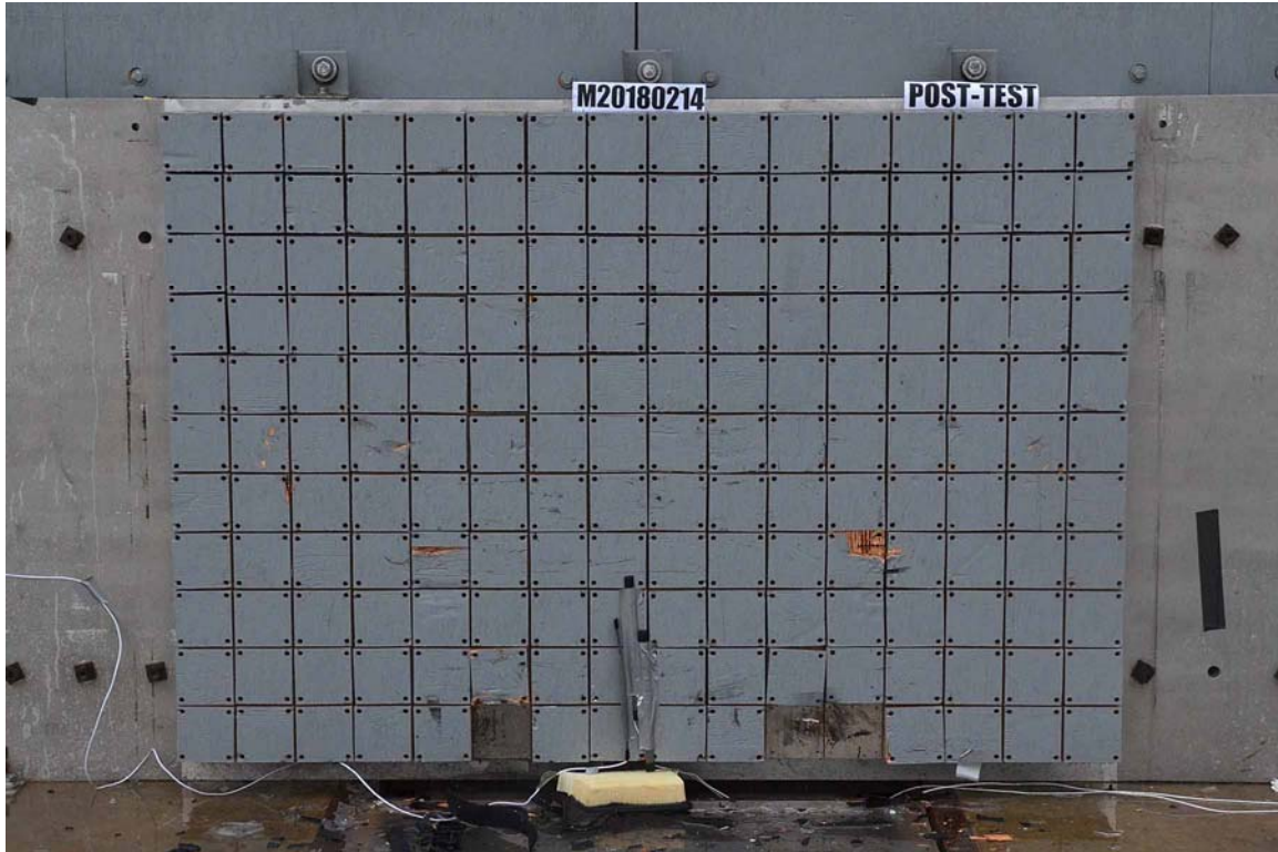
FIGURE 3. Post-Test Load Cell Wall
