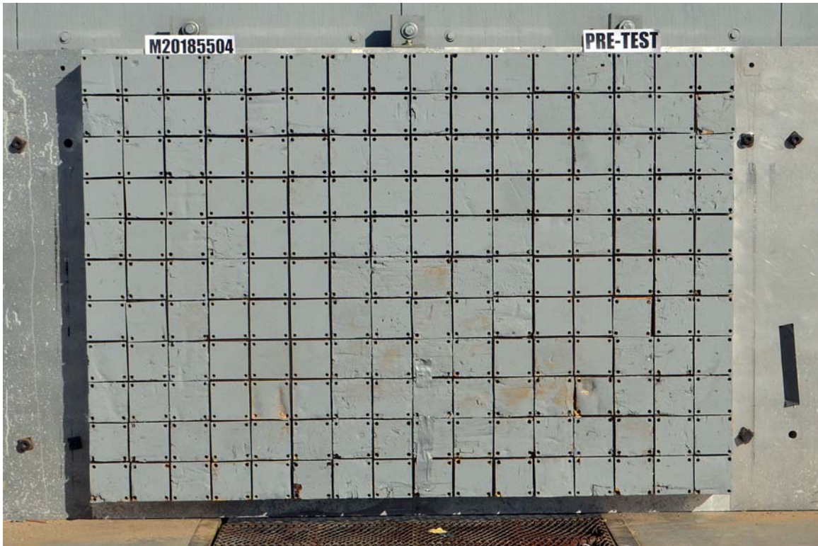
FIGURE 2. Pre-Test Load Cell Wall
