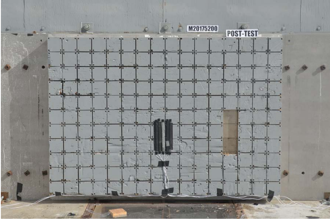
FIGURE 3. Post-Test Load Cell Wall
