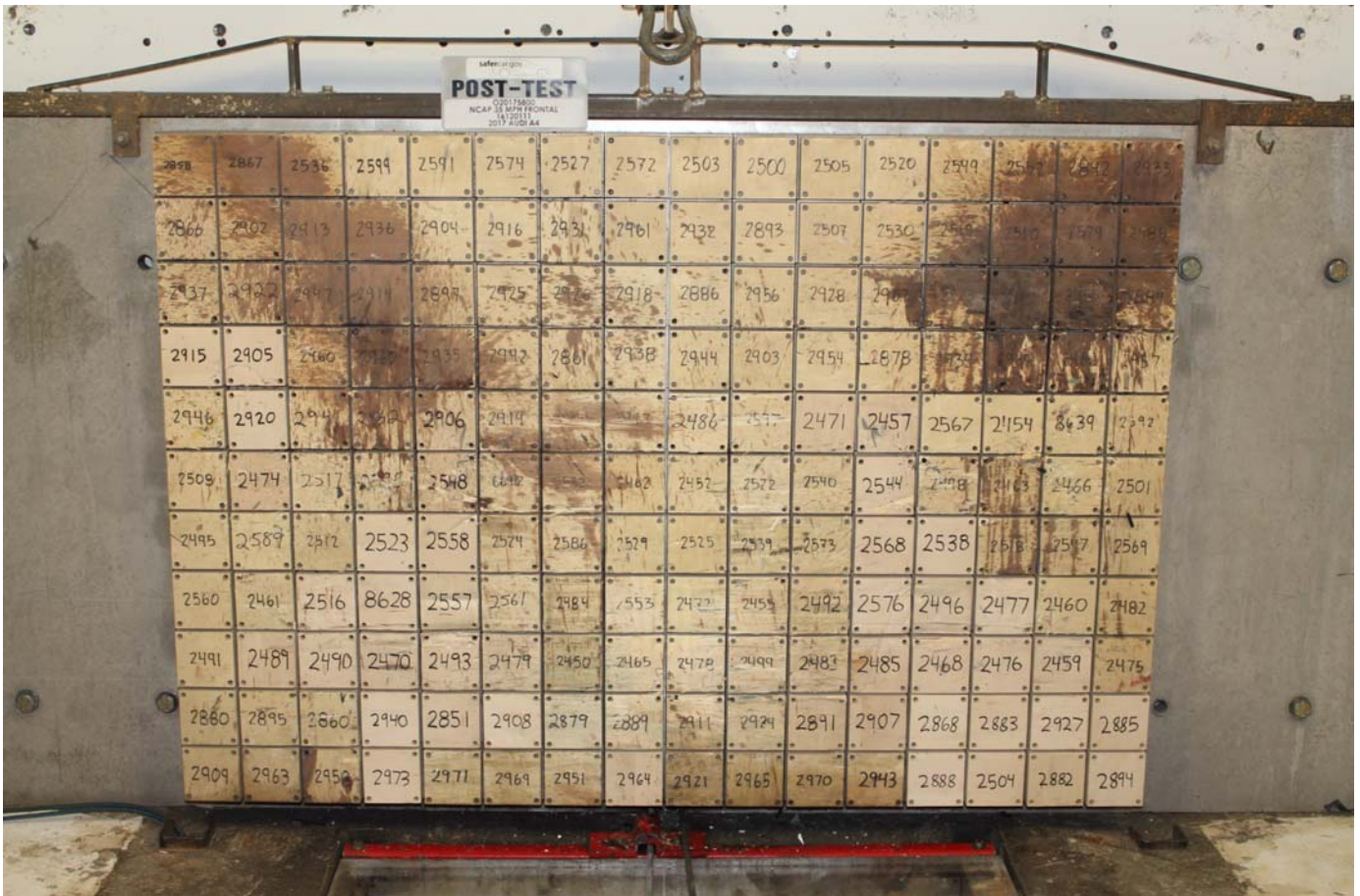
Photo No. 003 - Post-Test Load Cell Wall
